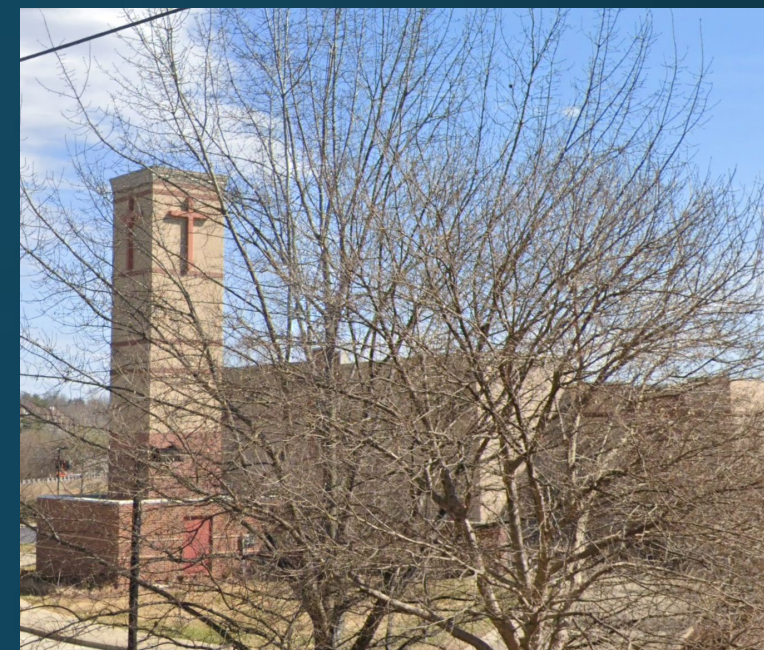
55-foot tower, Lewisburg Pk
