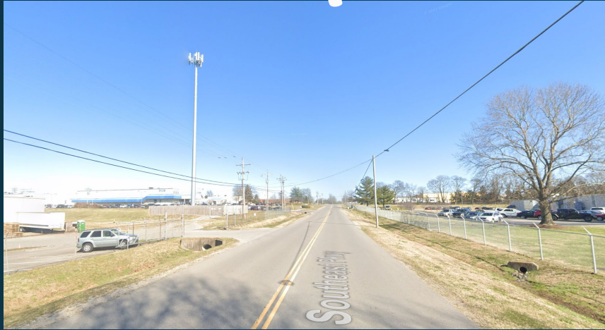
160-foot tower , Southeast Parkway
