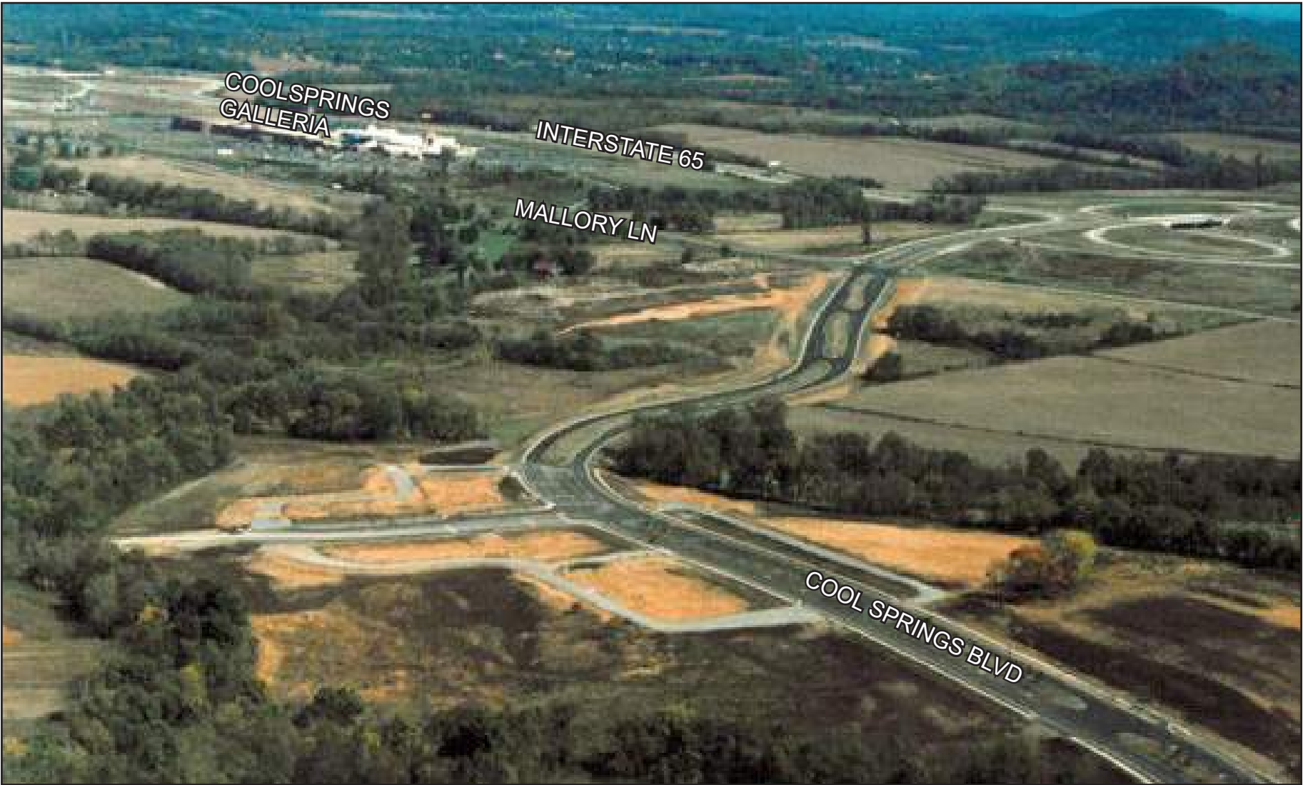
Cool Springs Boulevard, constructed to connect Mack Hatcher Parkway to the mall and the interstate.
