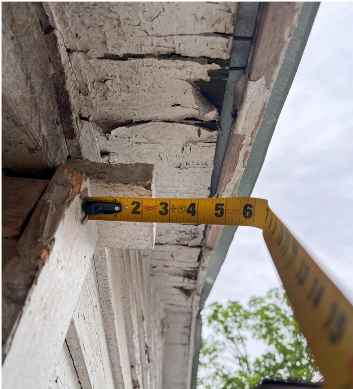
3 EXISTING ROOF OVERHANG @ REAR
