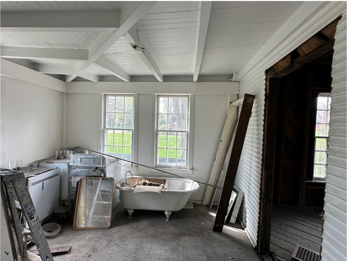
INTERIOR OF EXISTING ENCLOSED FRONT PORCH
