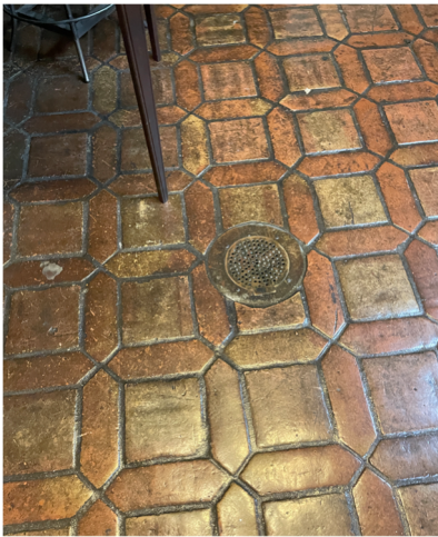
Original Stone Tile Walkways
