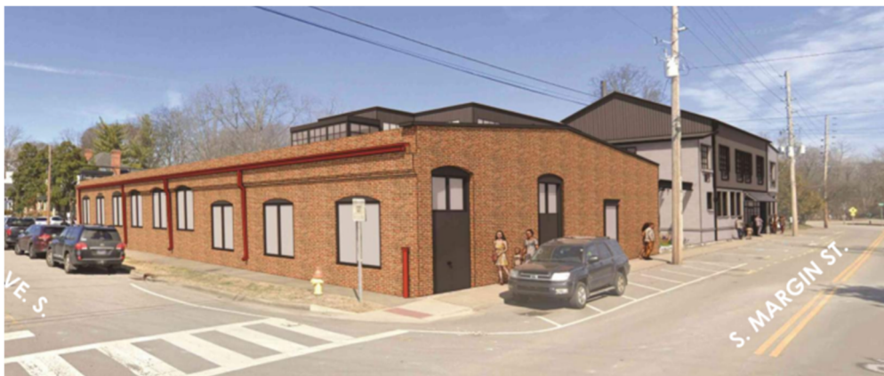
View from corner of 2 nd & Margin – addition is just visible over the top of the Icehouse
