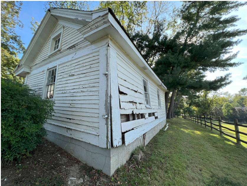
GARAGE RIGHT SIDE AND REAR
