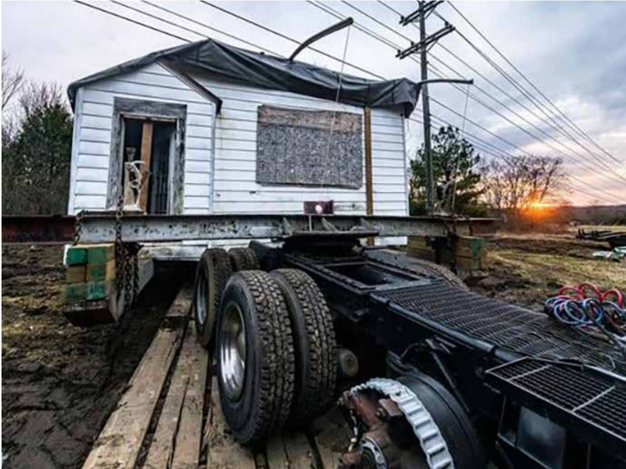
The last remaining Rosenwald School in Williamson County has been moved from its previous location in Spring Hill to the Franklin Grove Estate and Gardens in downtown Franklin. The Heritage Foundation of Williamson County organized the move of the Lee-Buckner School to the property they manage in Franklin with plans to restore, preserve, and transform the former school building in “an accessible and lasting monument to education and Black history.” The new, $35 million Franklin Grove Estate and Gardens broke ground in late 2023 with the goal of preserving historical structures from throughout Williamson County. It took just over two hours to move the school structure, witnessed by both community leaders and former students of the school. The Lee-Buckner School served children in the Rural Hill area of Williamson County from 1927 until it was closed amid desegregation in 1965. It served as a private residence until the 1990s.
