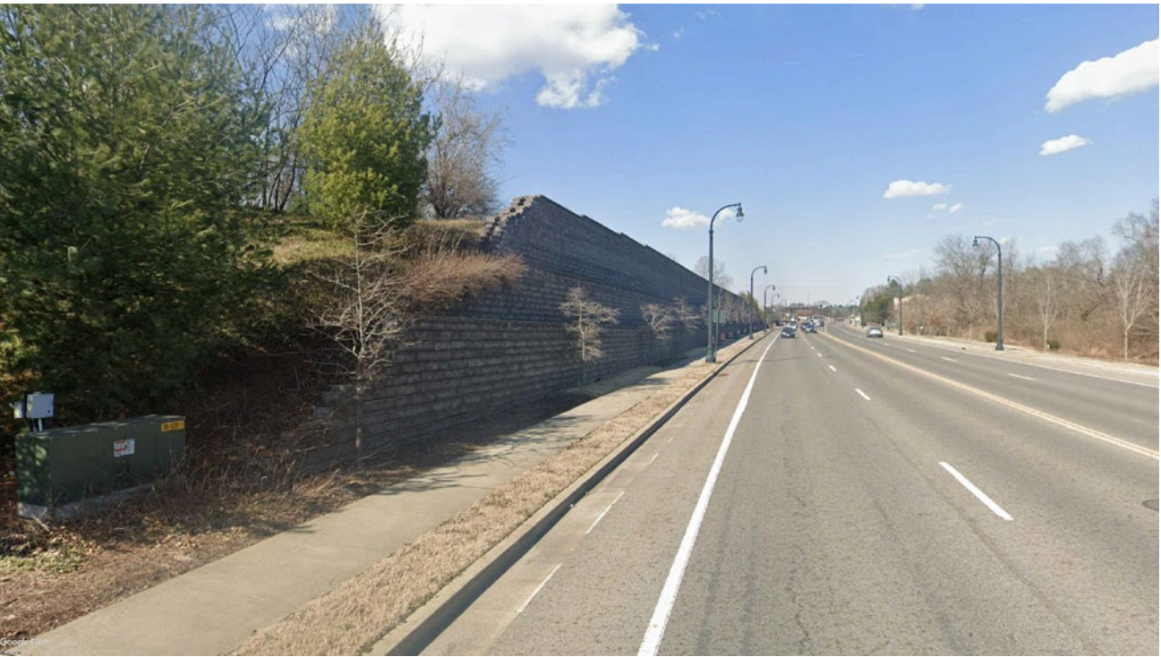
EXISTING CONDITION: 25' RETAINING WALL ALONG 5TH AVE N FRONTAGE
