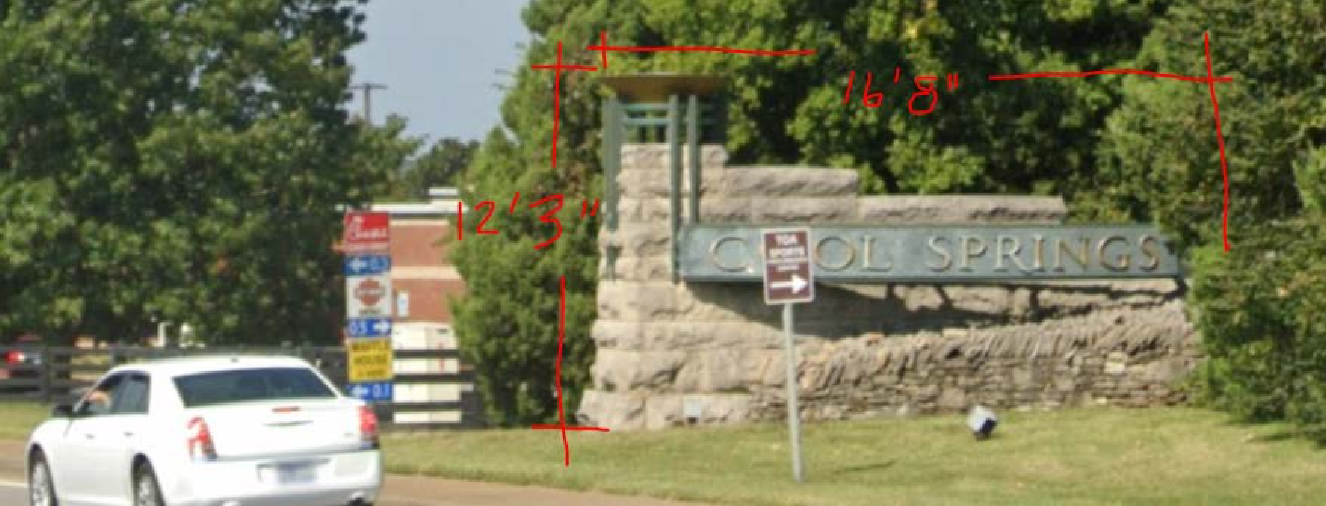
EXISTING CONDITIONS - PRECEDENT IMAGE
