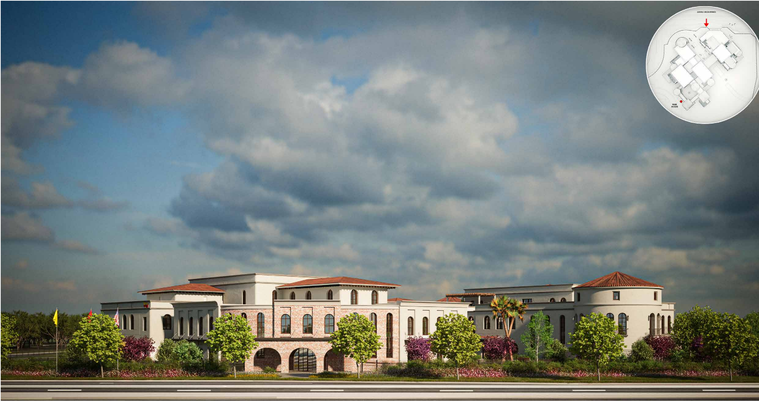
OFFICE - NORTH FACADE
