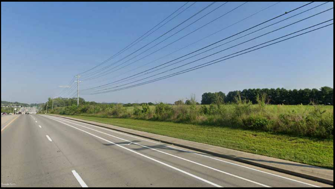
EXISTING OVERHEAD ELECTRIC LINES TO BE BURIED ALONG GOOSE CREEK BYPASS
