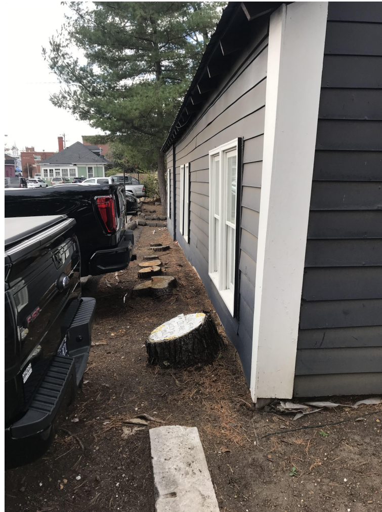
EAST (SOUTHEAST FACADE)
