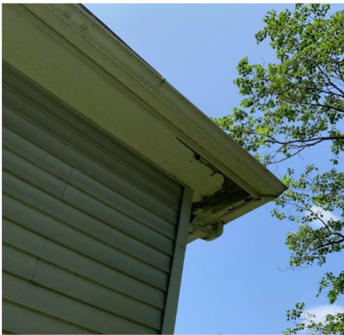
Image 17 & 18 - Severe deterioration at eave
