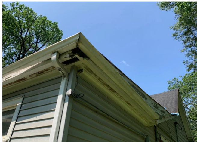
Image 17 & 18 - Severe deterioration at eave
