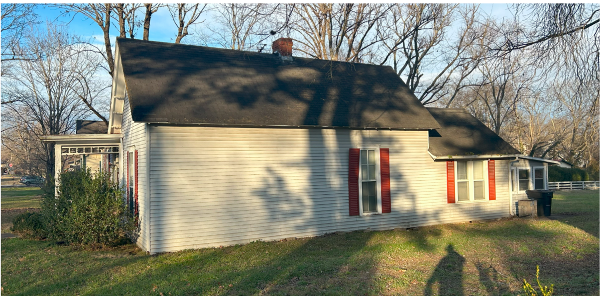
Image 2 - Right side (from standing at the front) view of the home
