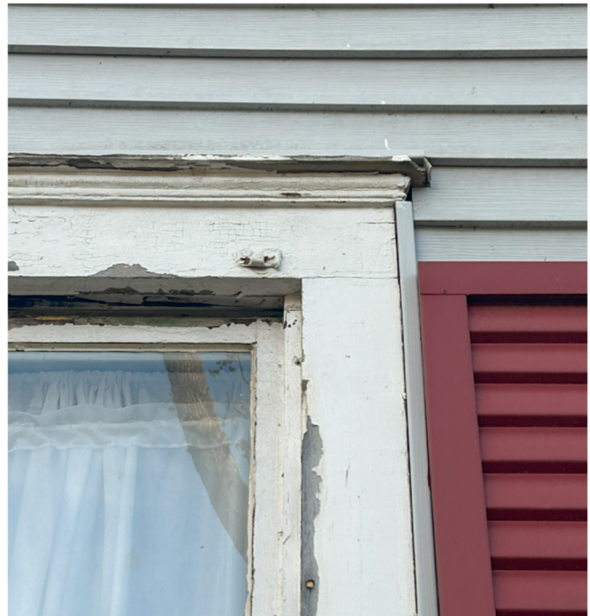
Images 9 & 10 - Vinyl siding & non-operable vinyl shutters have been added around window trim and poor detail has caused deterioration
