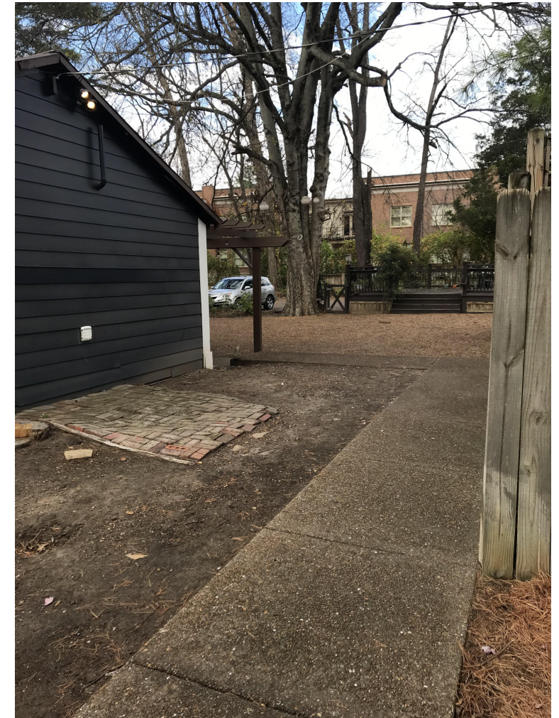
EAST (NORTHEAST FACADE)
