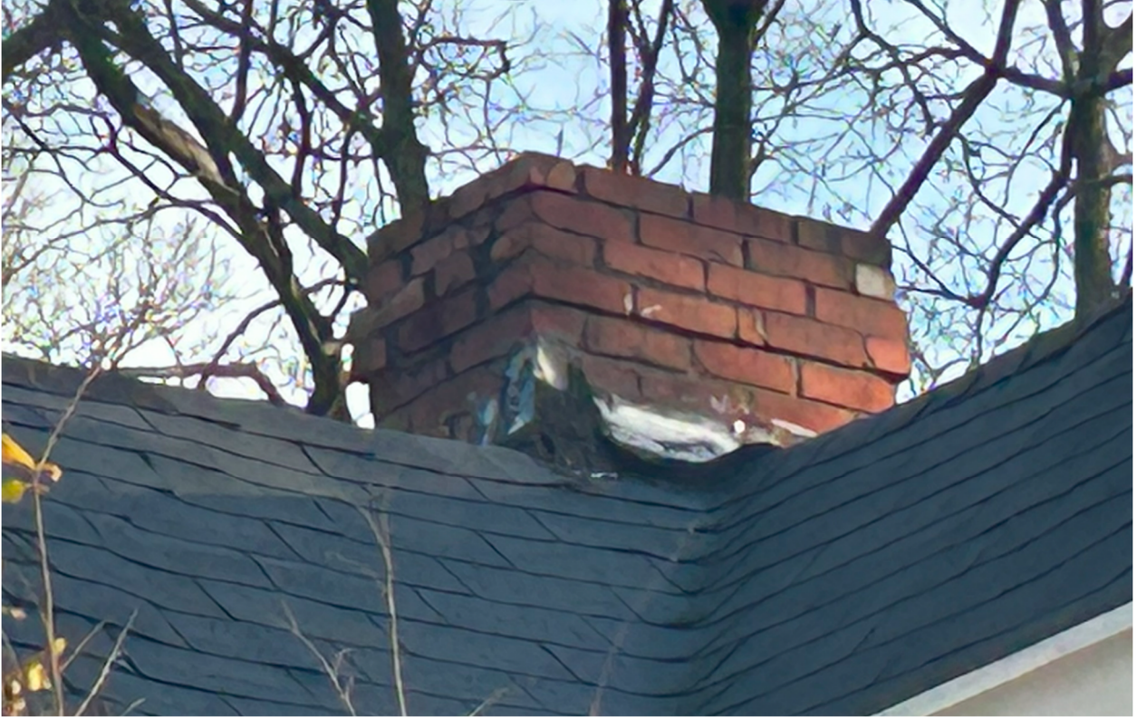
Image 16 - No distinctive brick detailing at chimney
