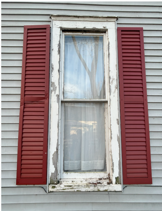
Images 9 & 10 - Vinyl siding & non-operable vinyl shutters have been added around window trim and poor detail has caused deterioration
