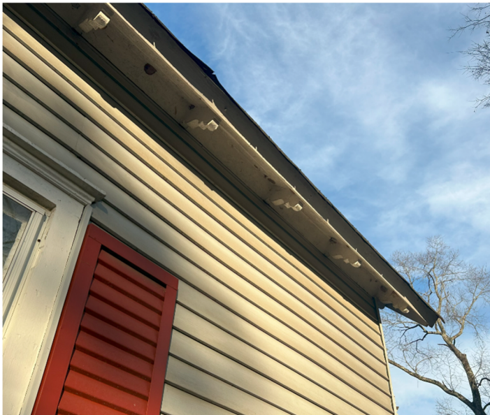
Images 12 & 13 - Left image: Original rafter extensions with scroll detail Right: rafter extensions at rear addition (no scrolled detail)
