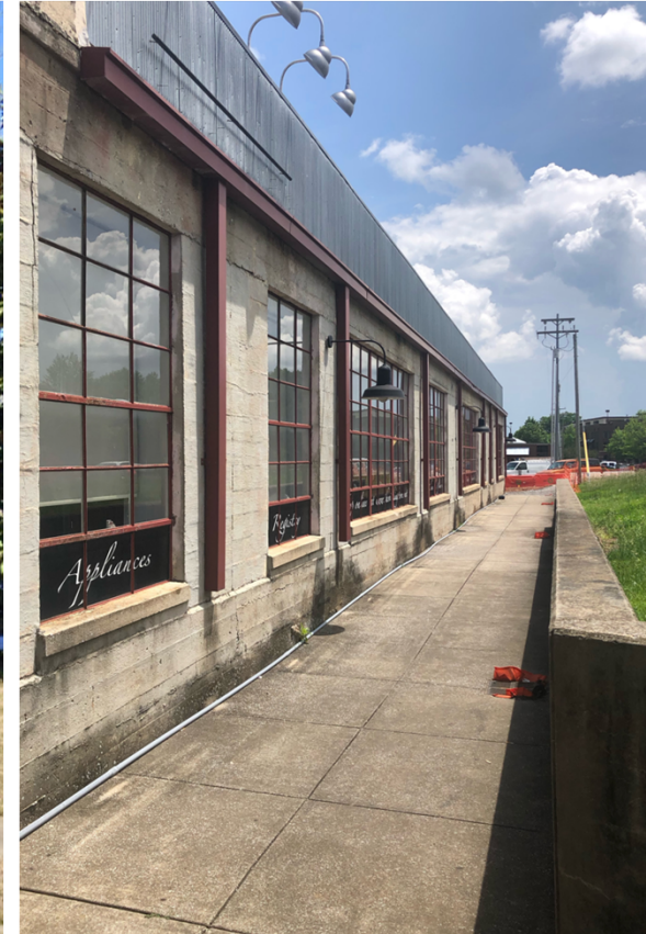
PHOTO OF EXISTING MECHANICAL SCREEN, BUILDING 13 EAST OF PROJECT LOCATION
