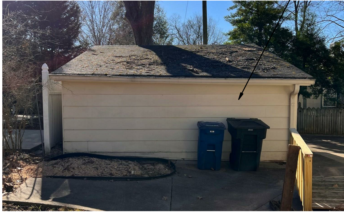
CARRIAGE HOUSE LEFT SIDE
