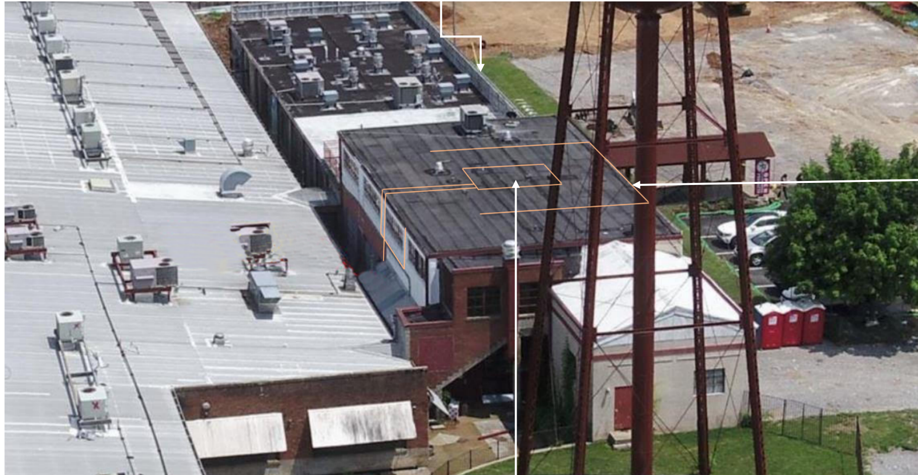
AERIAL VIEW OF ROOF
