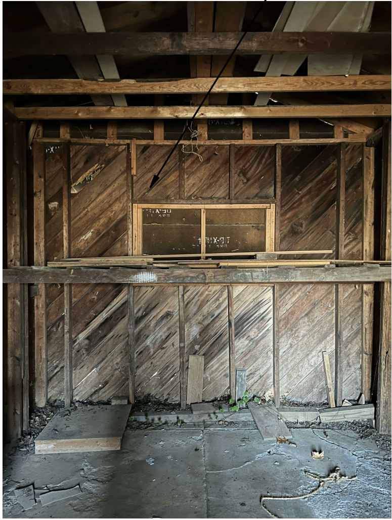
INTERIOR OF RIGHT PORTION OF CARRIAGE HOUSE
