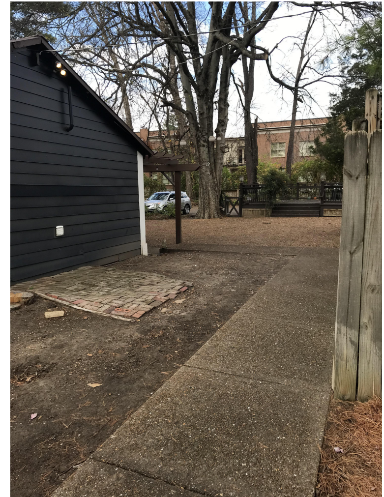
EAST (NORTHEAST FACADE)
