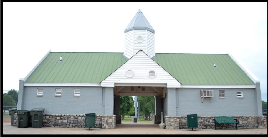
PK24008 - Fieldstone Concession and Pavilion Rehabilitation
