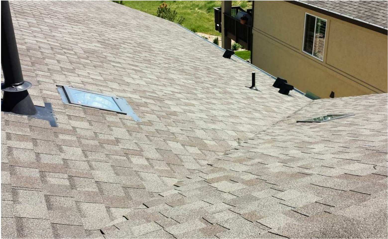
OPTION 1: FLAT PANEL SUN TUNNEL
