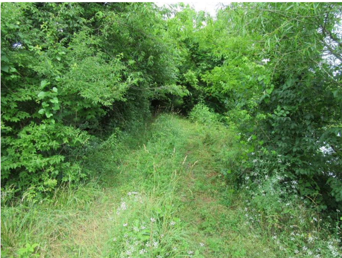
Photo No. 2: Crest viewed from left abutment.
