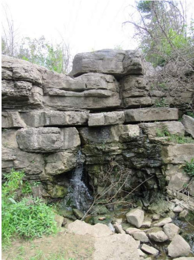
Photo No. 21: Seepage through bedrock at downstream end of spillway discharge channel.
