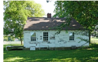
2 SOUTH WORKER HOUSE 1
