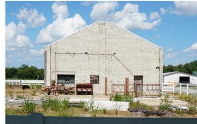
1 EAST POWER STATION
