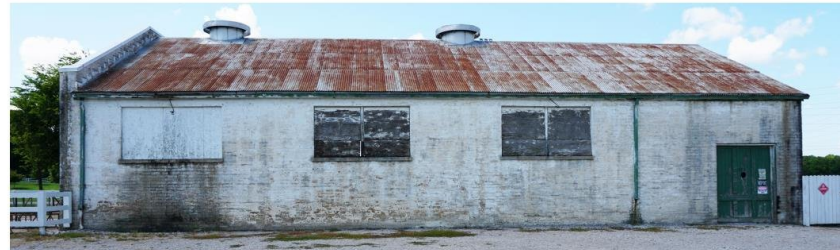
3 NORTH POWER STATION
