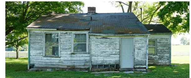
8 SOUTH WORKER HOUSE 2
