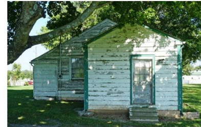
5 EAST WORKER HOUSE 2
