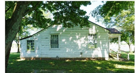
3 EAST WORKER HOUSE 1
