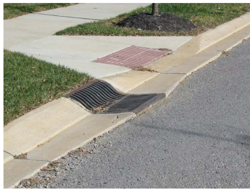
Rollover curb with grate transition
