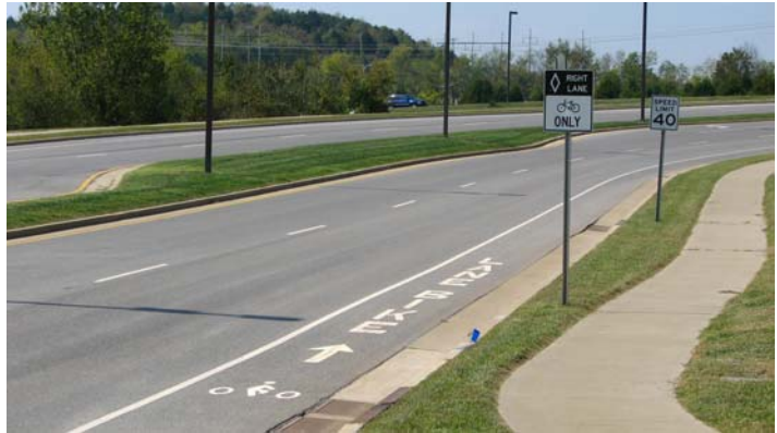
Typical bike lane with signing and markings
