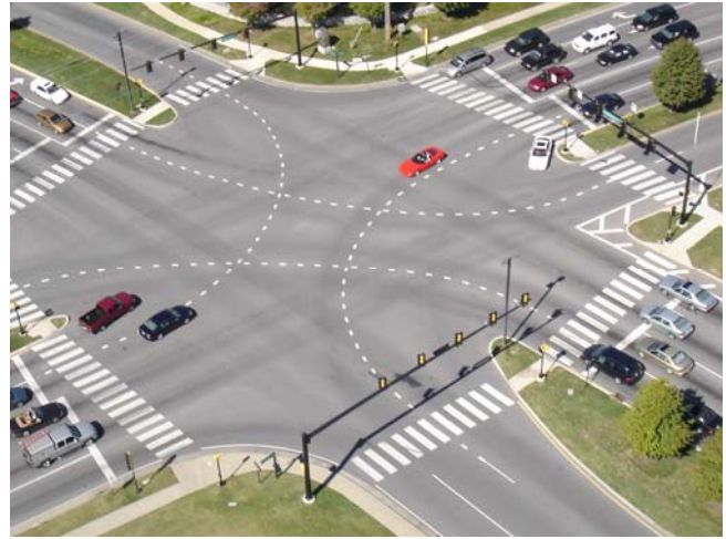
Channelization at intersection
