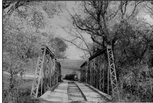
B. Bridge over Harpeth River at McGavock's Ford ca.1972 leading to Riverside, home of Dr. R.W. Billington, from Lewisburg Pike. Lcoals called it "Old Squeaky."
