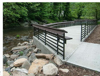
Accessible Fishing Piers
