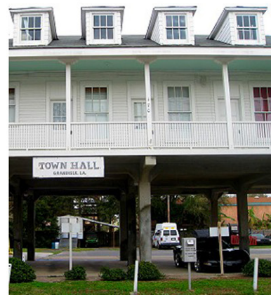
D. Building on piers
