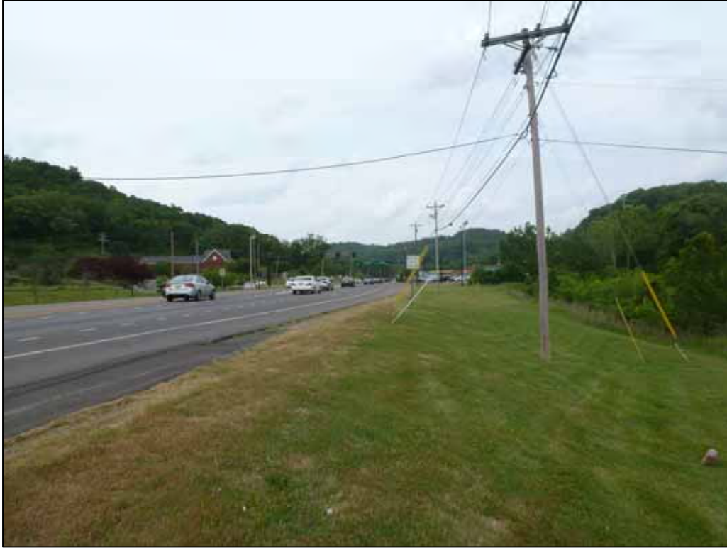
Northerly view along Franklin Road ROW
