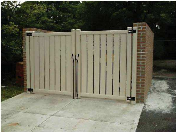
BRICK TRASH ENCLOSURE EXAMPLE
