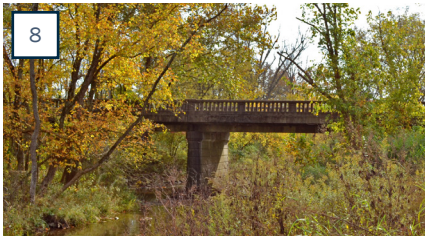
View of Mayes Creek Bridge
