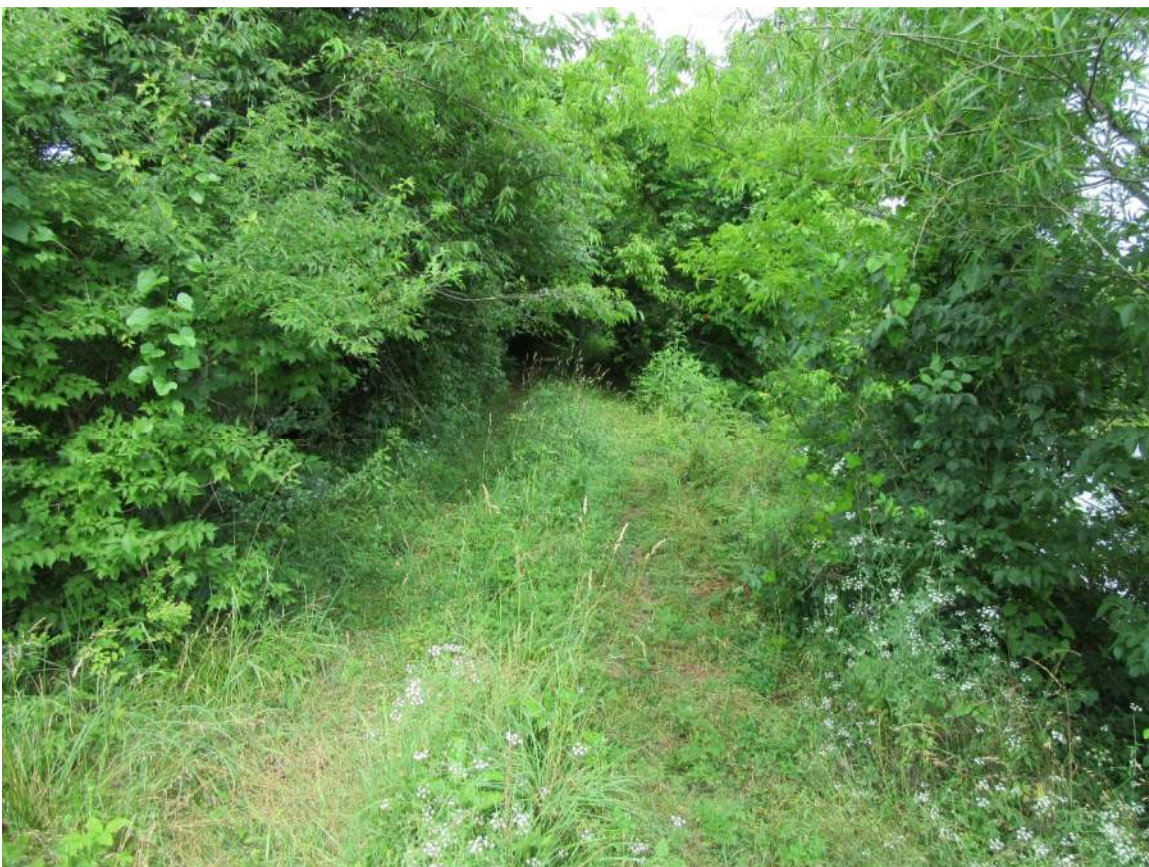
Photo No. 2: Crest viewed from left abutment.
