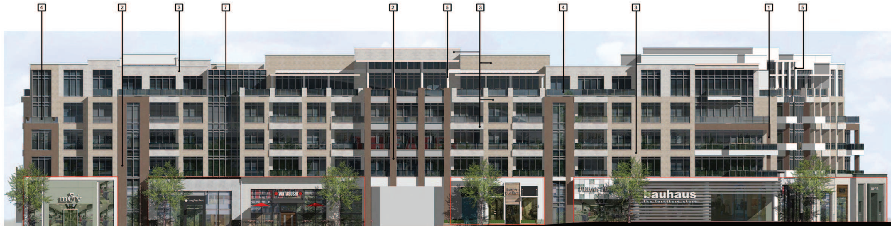
TYPICAL RESIDENTIAL BUILDING
