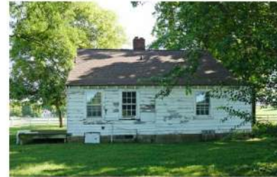
2 SOUTH WORKER HOUSE 1
