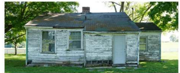
8 SOUTH WORKER HOUSE 2
