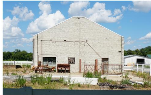
1 EAST POWER STATION
