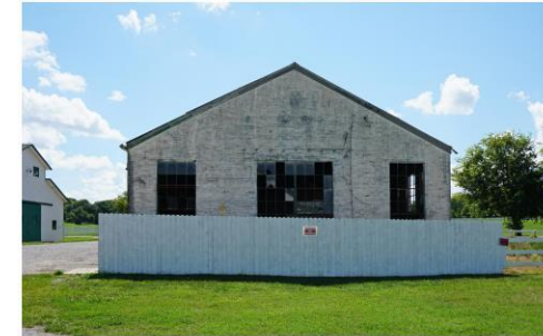
2 WEST POWER STATION
