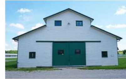
2 SOUTH MAIN BARN
