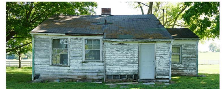
8 SOUTH WORKER HOUSE 2
