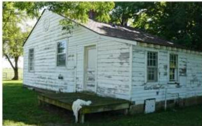
4 WEST WORKER HOUSE 1
