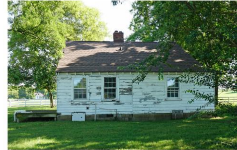
2 SOUTH WORKER HOUSE 1
