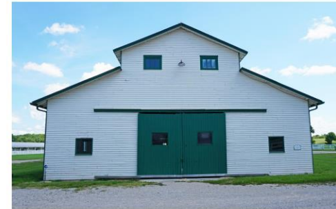
2 SOUTH MAIN BARN
