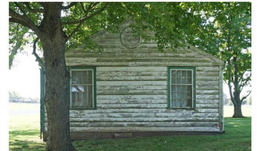
6 WEST WORKER HOUSE 2
