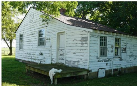
4 WEST WORKER HOUSE 1
