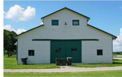
1 NORTH MAIN BARN
