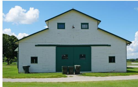
1 NORTH MAIN BARN
