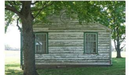
6 WEST WORKER HOUSE 2
