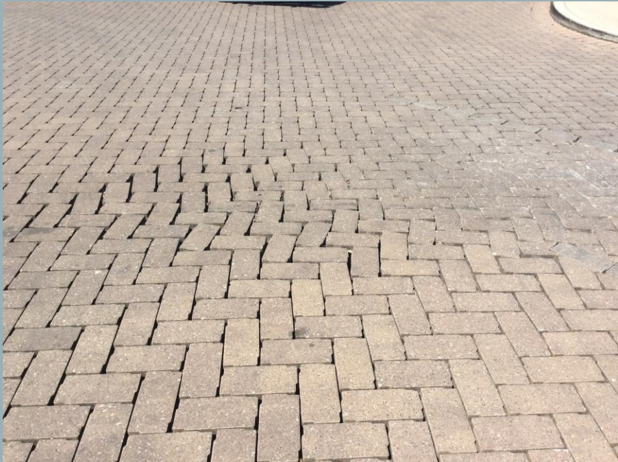
First Bank @ Five Points: Reinstall permeable pavers
