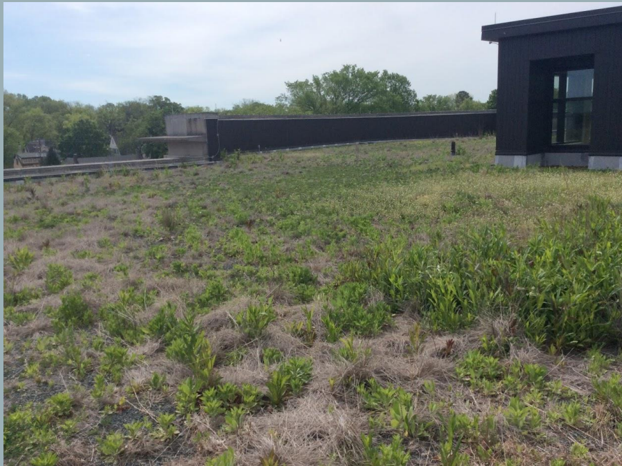
Green roof at Police Headquarters
