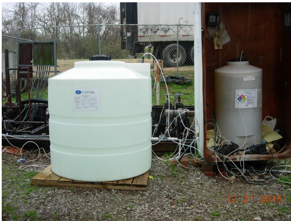
Captor de-chlorination solution tank (left) & chlorine solution tank (right)
