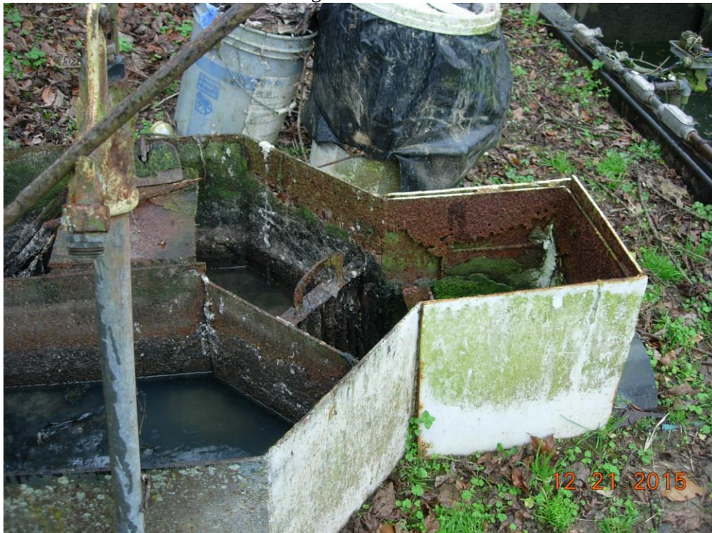
Severe corrosion of bar screen structure & metal walls breaking apart
