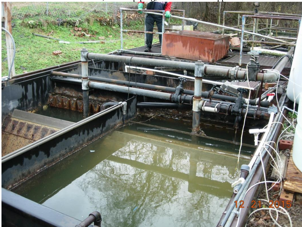
Corroded filter structure & weir troughs, & chlorine feed lines
