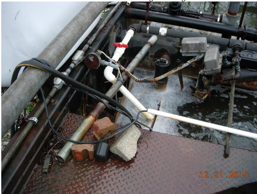
Corroded pipes broken off, emergency overflow weir box severely corroded, piping held up with broom handle & galvanized pipe, wiring deteriorated, extension cords run across basin
