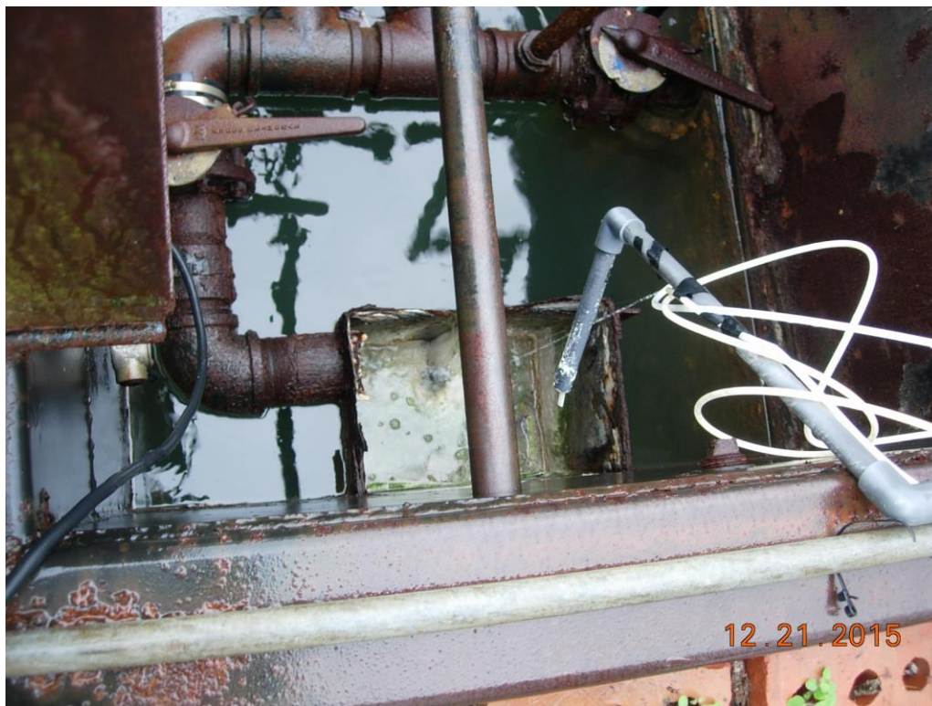
Corroded effluent weir box, Captor de-chlorination feed point, effluent discoloration in weir box
