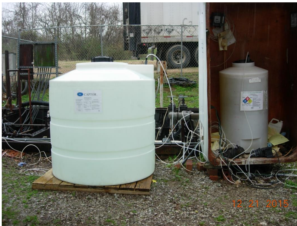
Captor de-chlorination solution tank (left) & chlorine solution tank (right)
