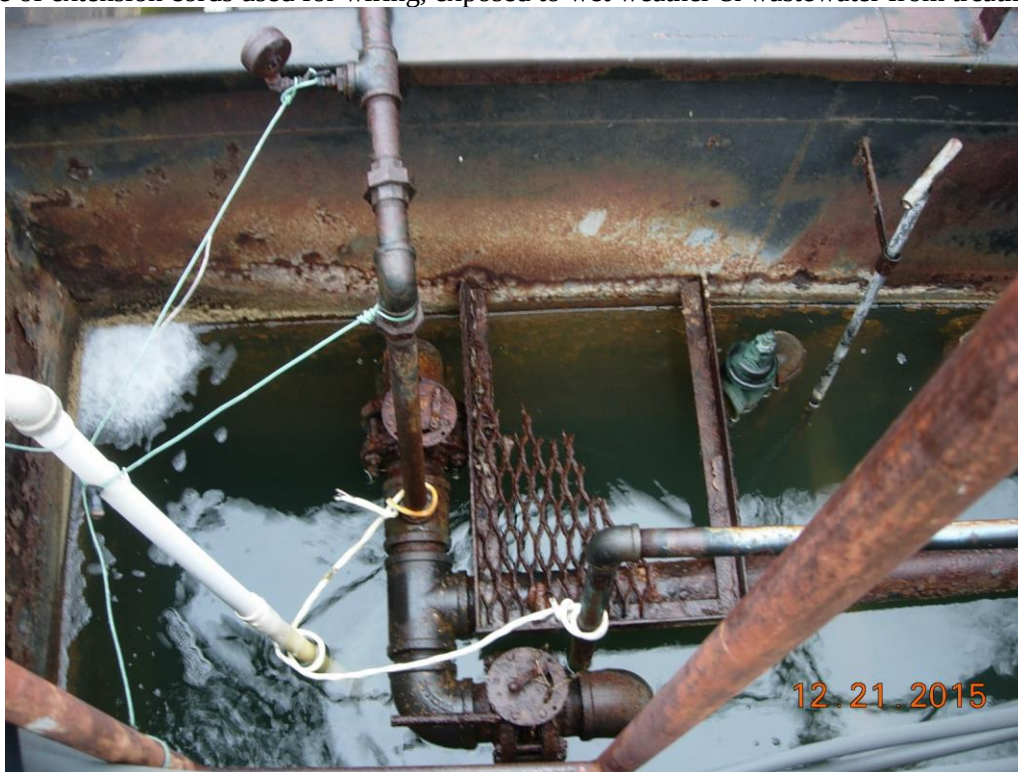
Corroded access platform & piping, makeshift piping for aeration in final effluent chamber
