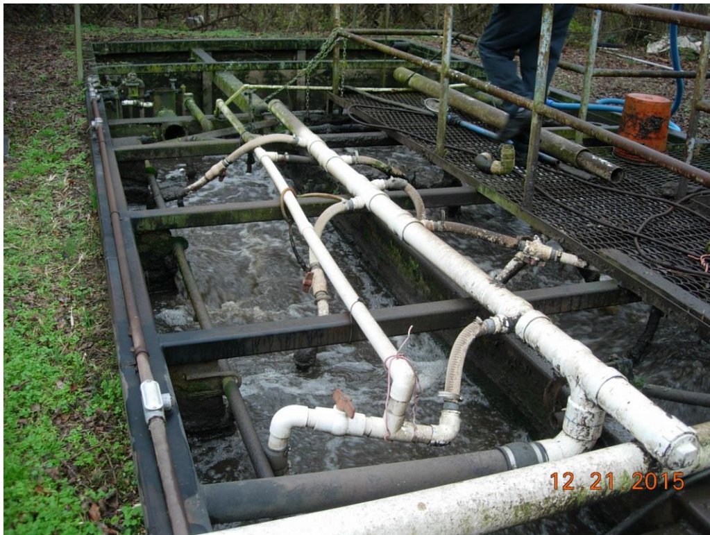
Aeration basin, PVC pipe & flexible hose replacing corroded & un-useable aeration lines
