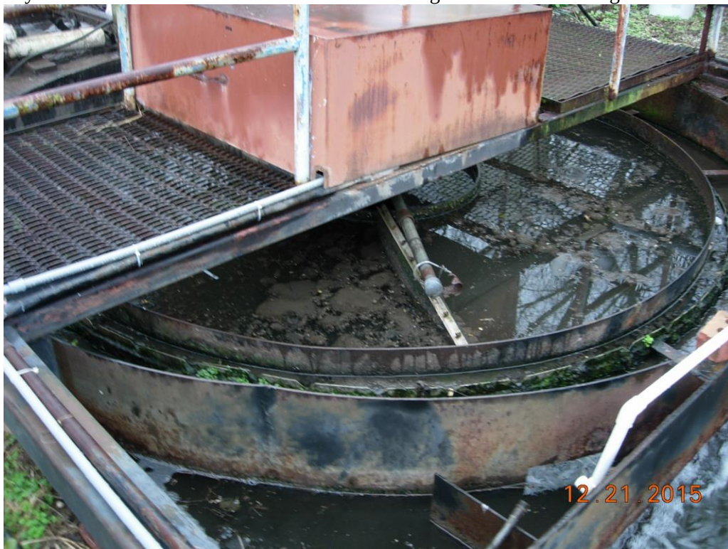
Rising solids in clarifier due to clogged sludge return line & inadequate treatment, surface skimmer broken & ineffective
