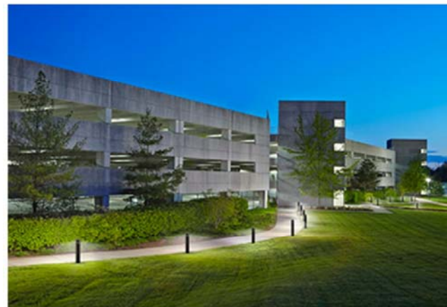
Bollard Lights (Type F) (Mounted at Grade)
