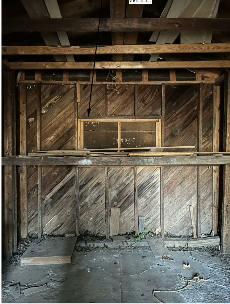
INTERIOR OF RIGHT PORTION OF CARRIAGE HOUSE
