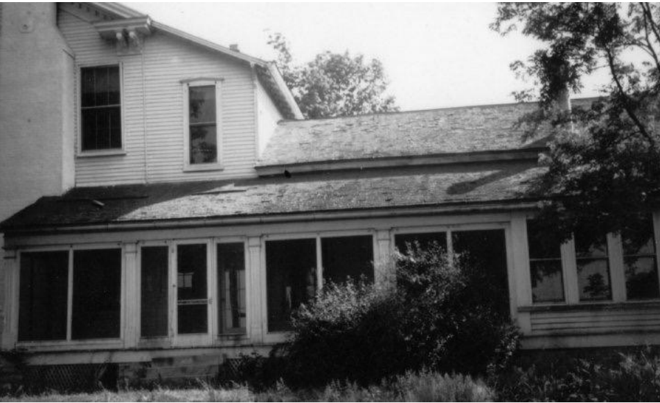
SIDE VIEW - EXISTING ADDITION THAT HAS BEEN DEMOLISHED
