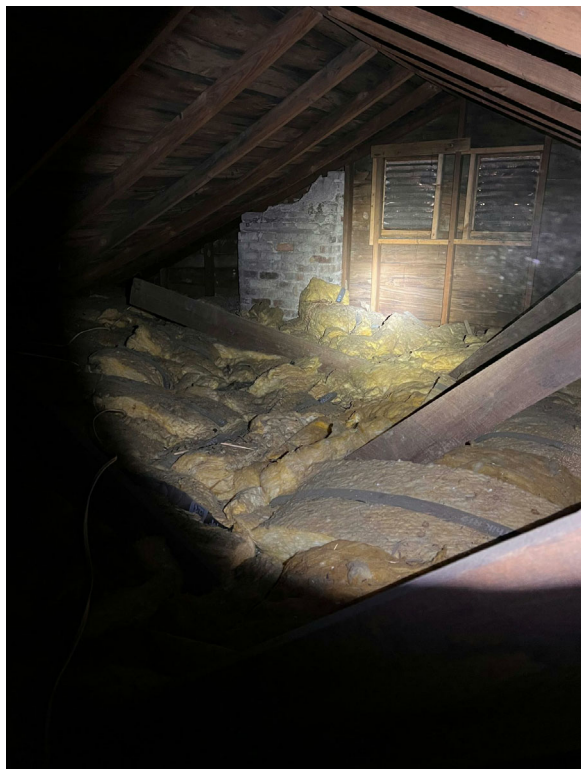
EXISTING CHIMNEY IN ATTIC SHOWING BRICK
