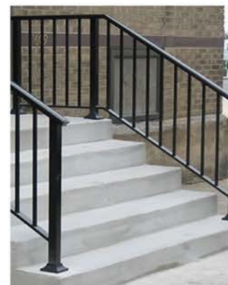
METAL RAILINGS AND CONCRETE STEPS
