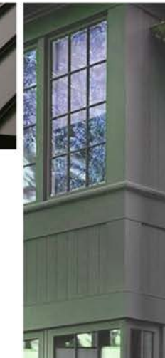
ALUMINUM COMPOSITE METAL AT BAY WINDOW
