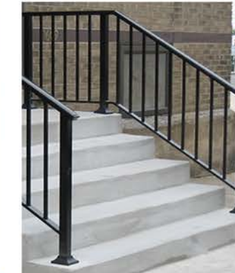
METAL RAILINGS AND CONCRETE STEPS
