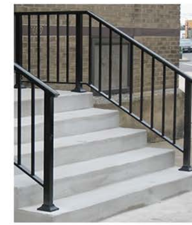
METAL RAILINGS AND CONCRETE STEPS
