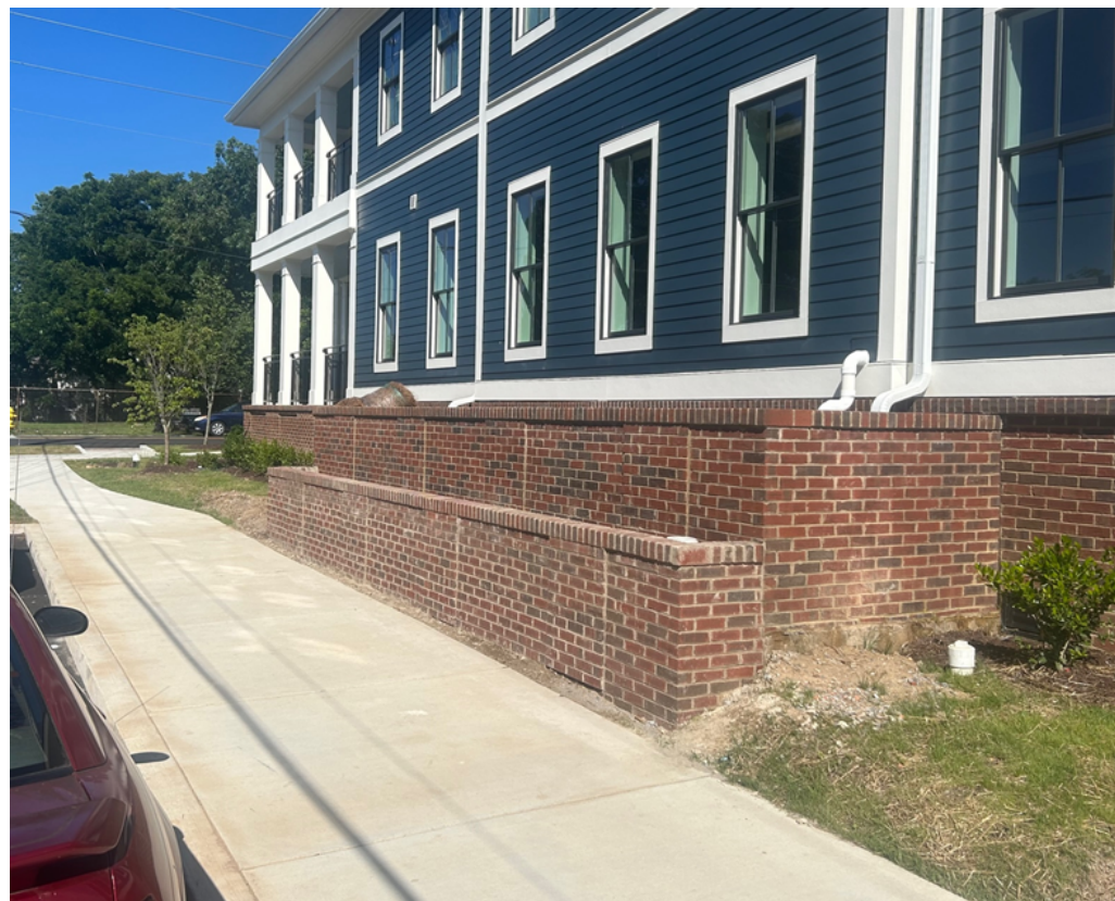
CURRENT VIEW FROM NORTH MARGIN LOOKING TOWARDS 4TH AVENUE
