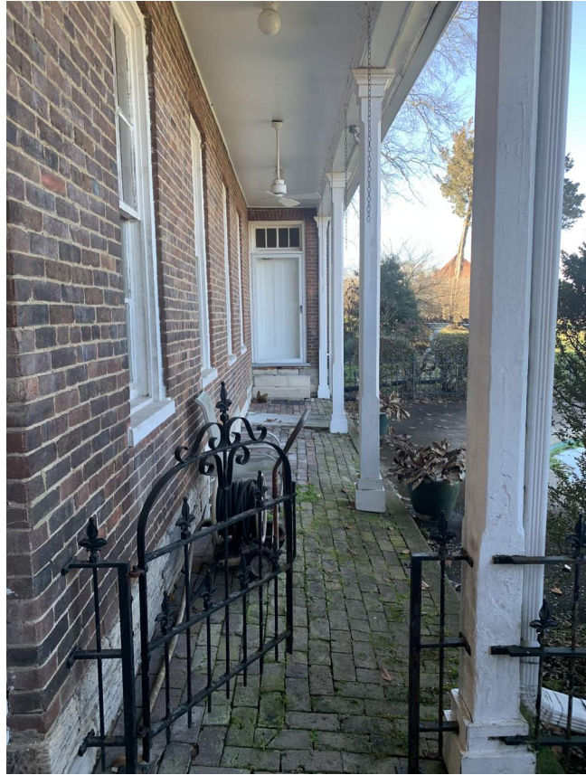
KITCHEN WING, REAR PORCH
