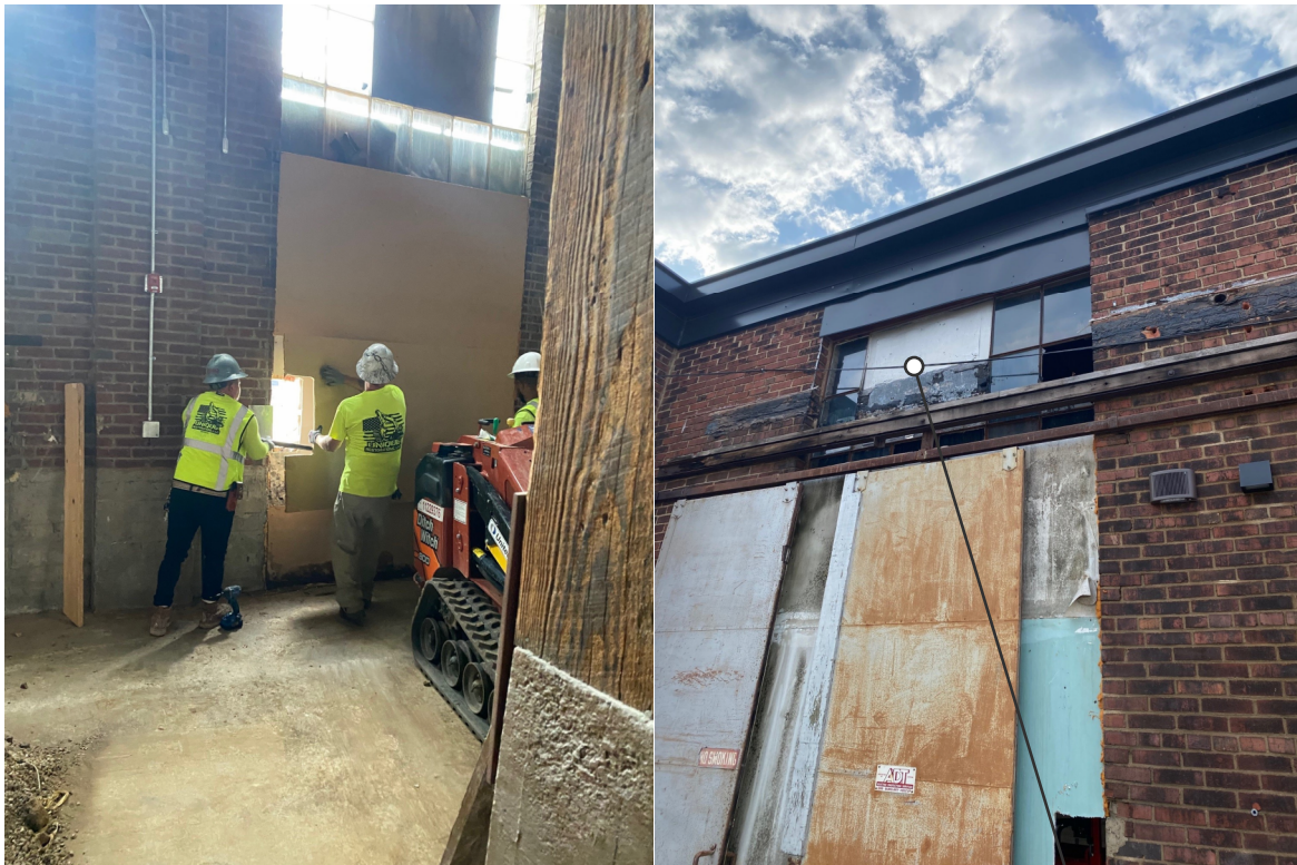
IMAGES DURING DEMOLITION TRANSOM A
