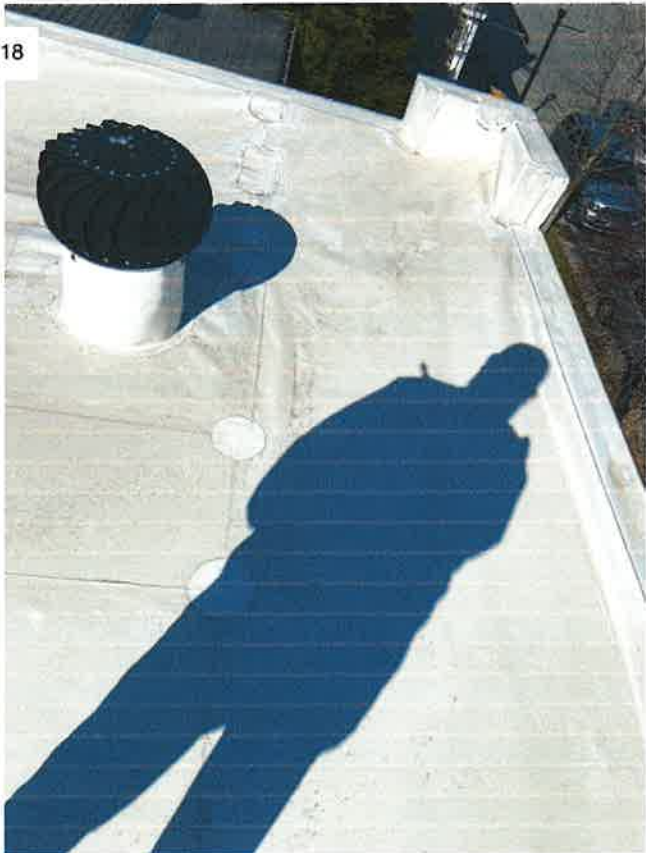
Project: 146 4th Ave S Date: 1/27/2023, 11:59am Creator: Donald Jakes
