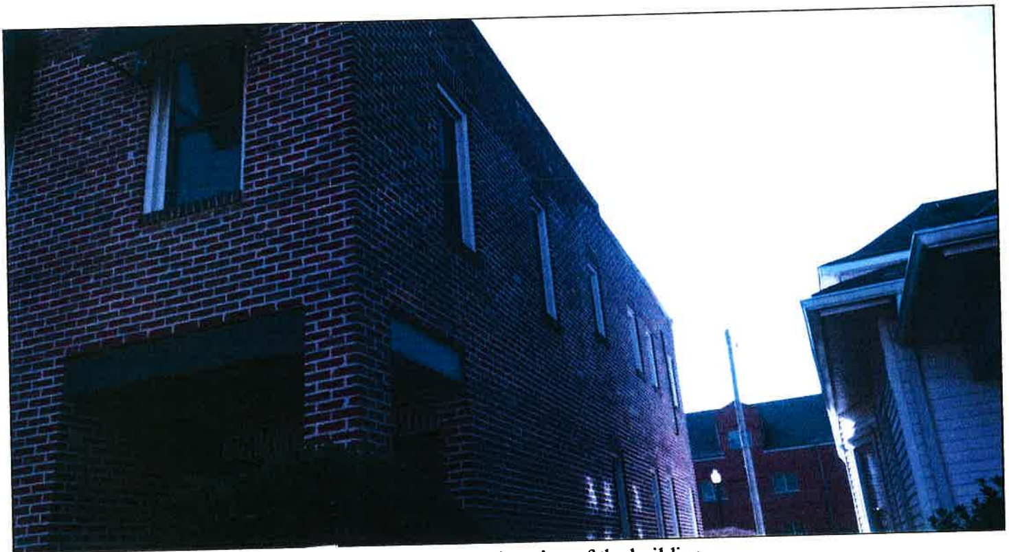
East (side) elevation of the building.
