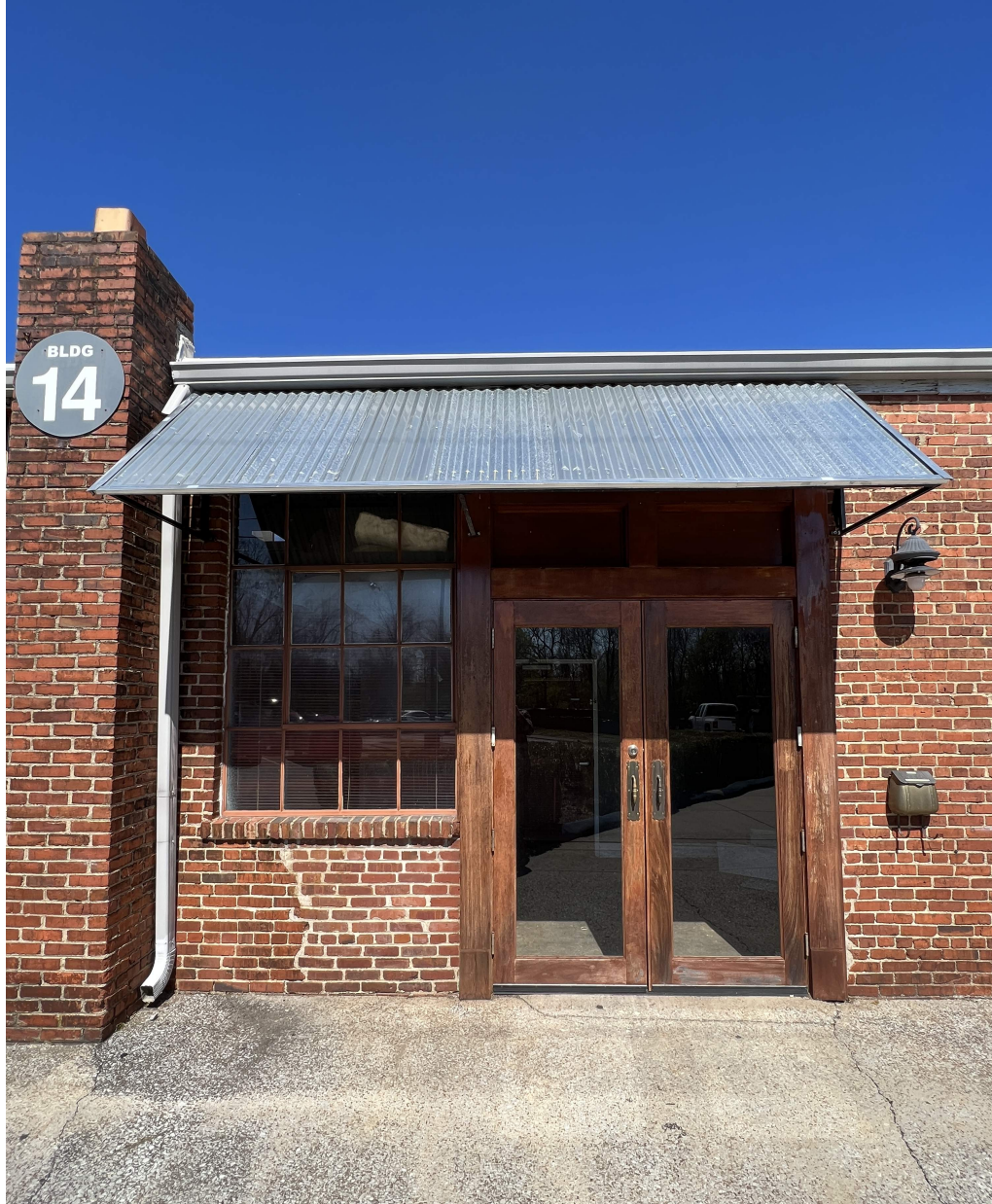
EXISTING PHOTO - ENTRY CANOPY
