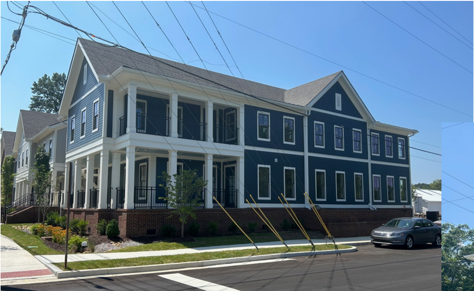
EXISTING CONDITION : VIEW FROM CORNER OF NORTH MARGIN AND 4TH AVE.
