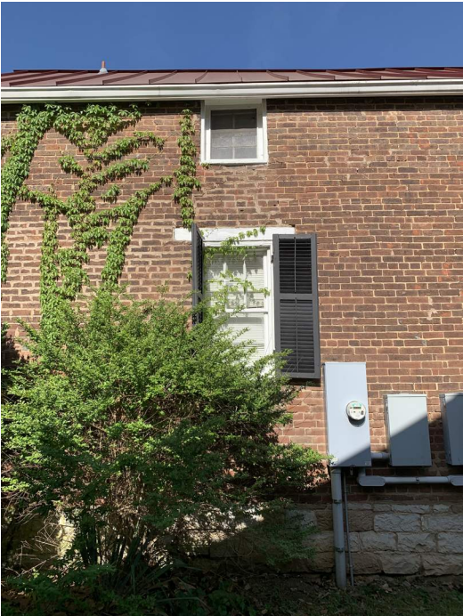
EAST WALL, OLD KITCHEN (FACING GARAGE)
