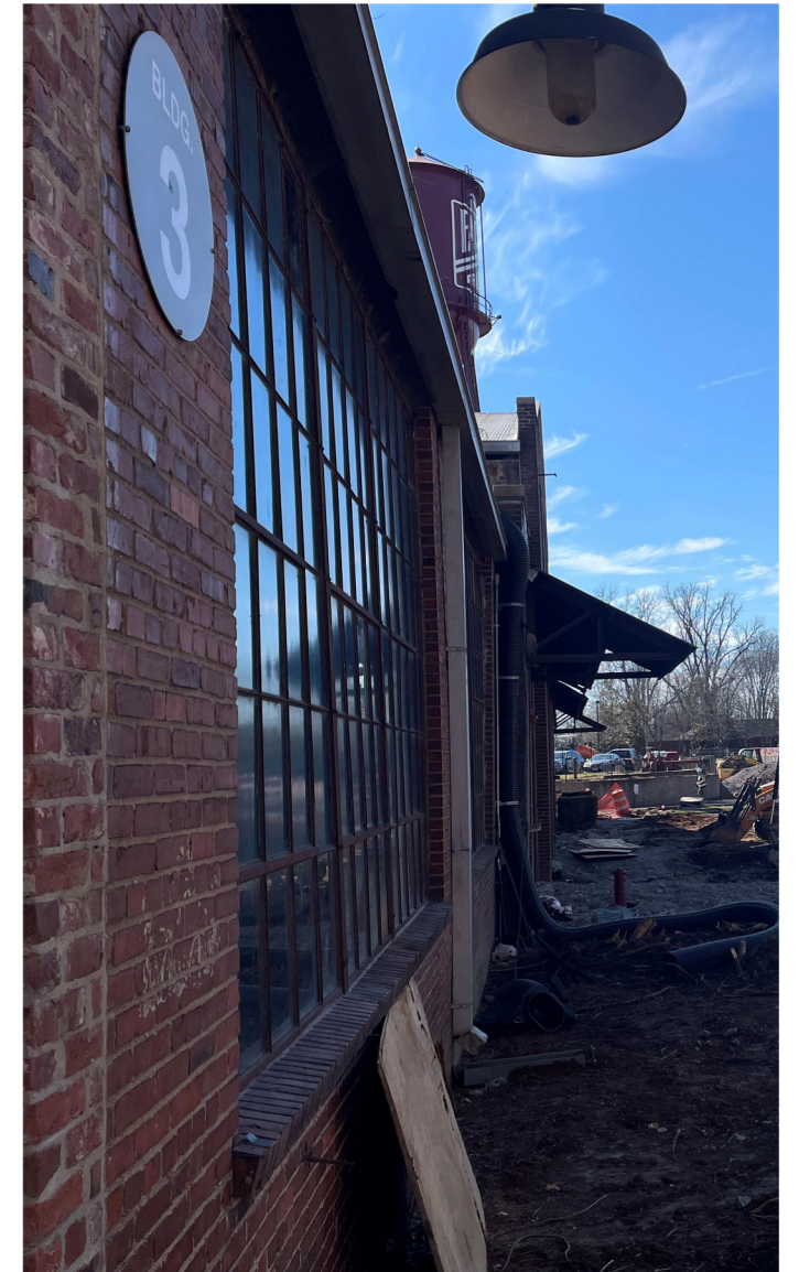
EXISTING CONDITIONS FOR CONTEXT:
