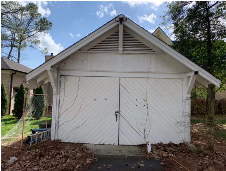
View of shed at the end of the driveway
