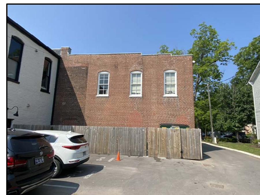
NEW MASONRY TO MATCH EXISTING COLOR AND TEXTURES - PROVIDE 'COMMON BOND' WITH 1TH ROW HEADER COURSE (TYP).
