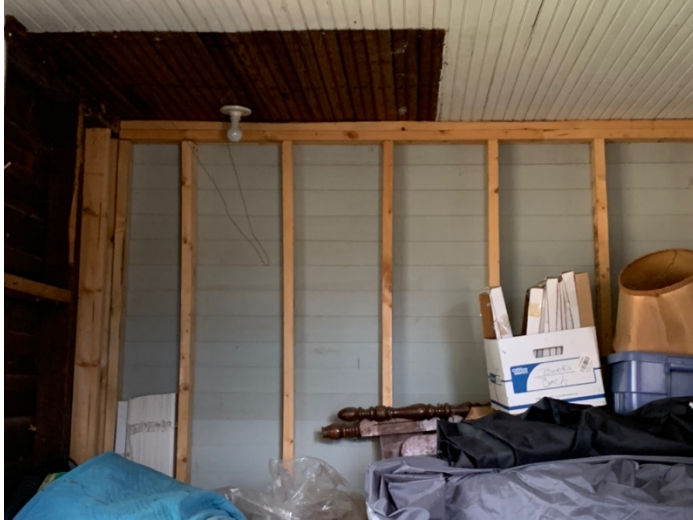
View of interior of shed showing new 'back wall'. This wall was reframed to shorten the original depth of the building in order to accommodate easement requirements between 425 Boyd Mill property line and Benelli Park development – Plot 1
