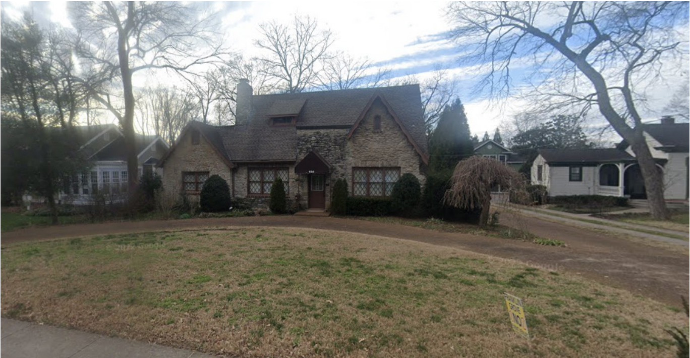
EXISTING HISTORIC STRUCTURE:: 116 LEWISBURG AVE, FRANKLIN, TN + Circular pull thru
