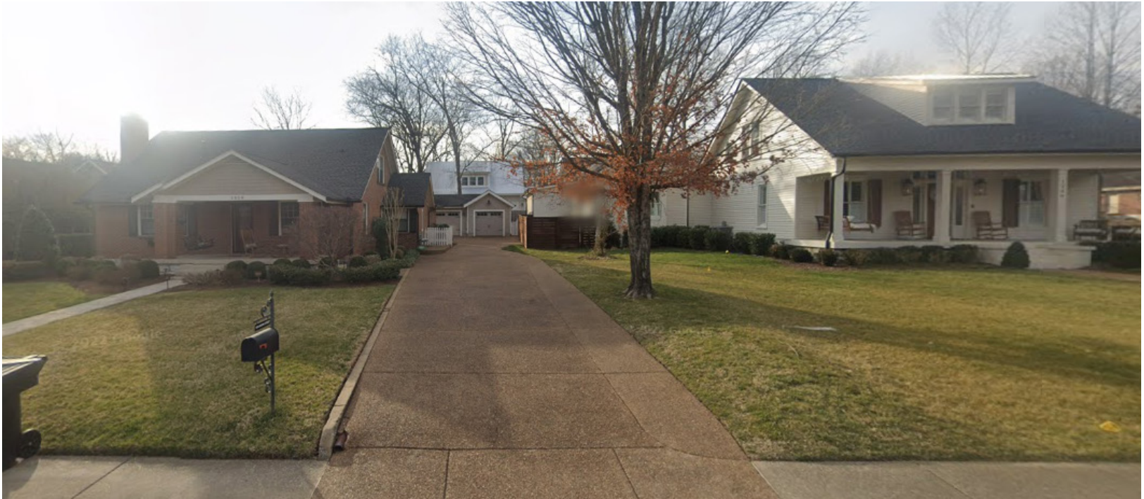
EXISTING HISTORIC STRUCTURE:: 1250 ADAMS STREET, FRANKLIN, TN + Front facing Garage
