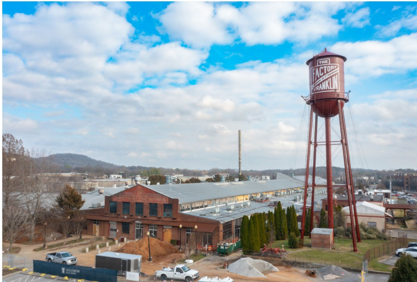
THE FACTORY - EXISTING PHOTO
