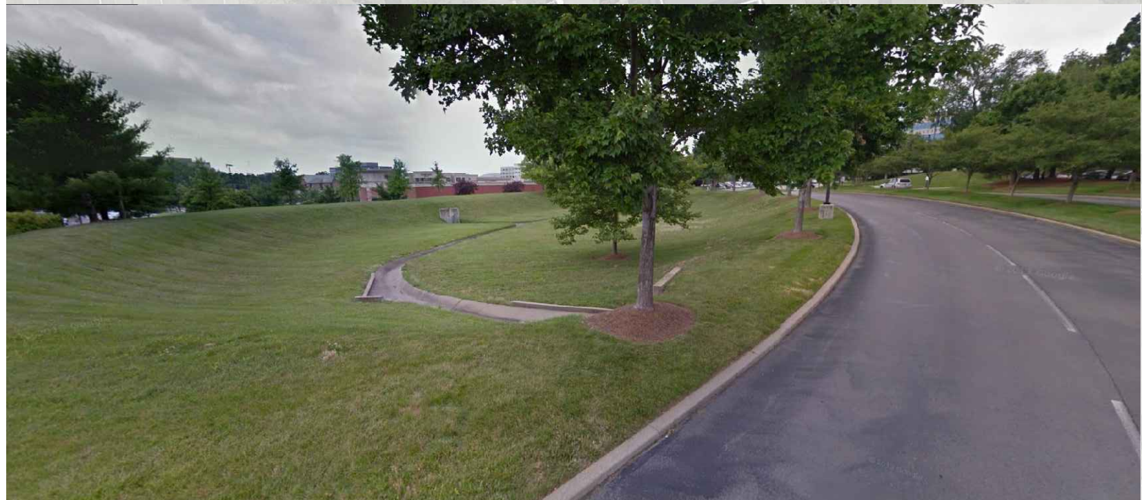
SE POND & OUTLET CONTROL STRUCTURE
