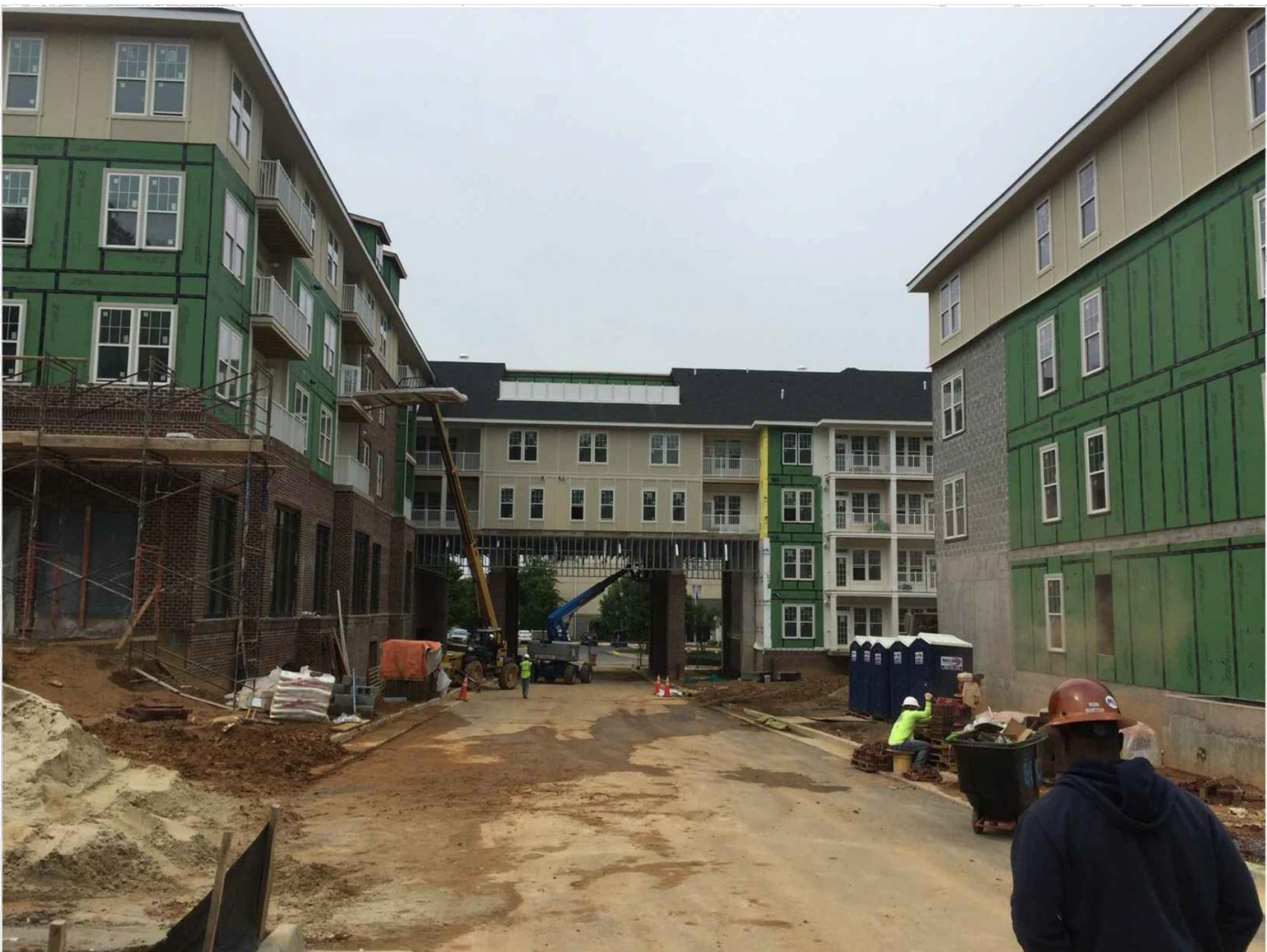
VIEW OF BRIDGE OVER PUBLIC STREET / FIRELANE
