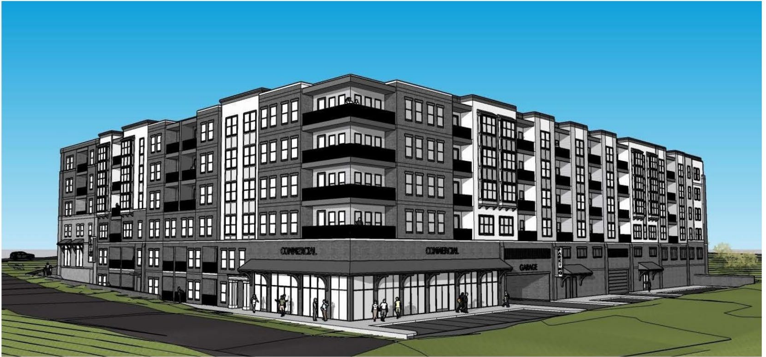
VIEW AT ACCESS ROAD AT BACK OF BUILDING
