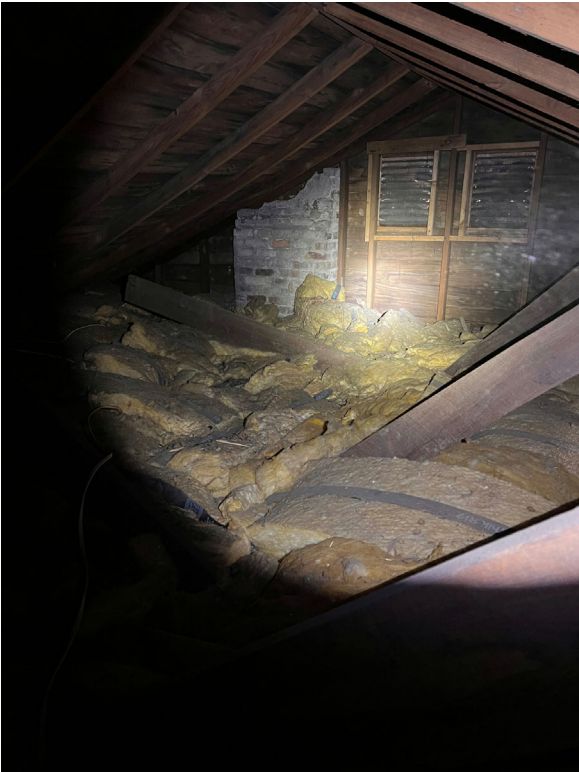
EXISTING CHIMNEY IN ATTIC SHOWING BRICK
