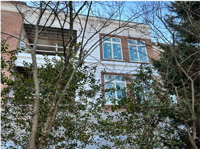
VIEW FROM ADJACENT PARKING LOT
