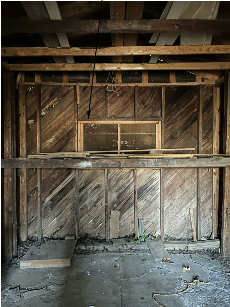
INTERIOR OF RIGHT PORTION OF GARAGE
