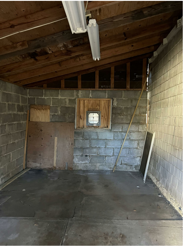
INTERIOR OF LEFT PORTION SHOWING SHAKE EXTERIOR
