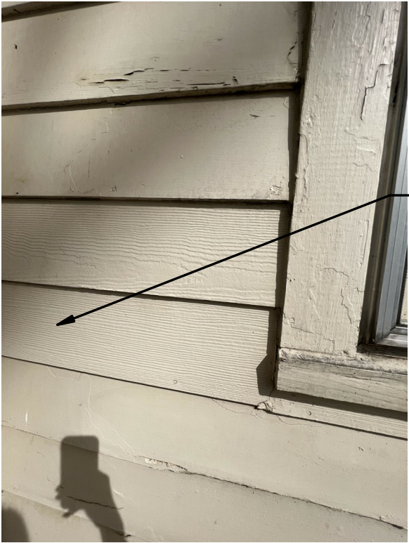
REAR ADDITION SOME BOARDS HAVE BEEN REPLACED WITH WOOD GRAIN HARDIE SIDING
