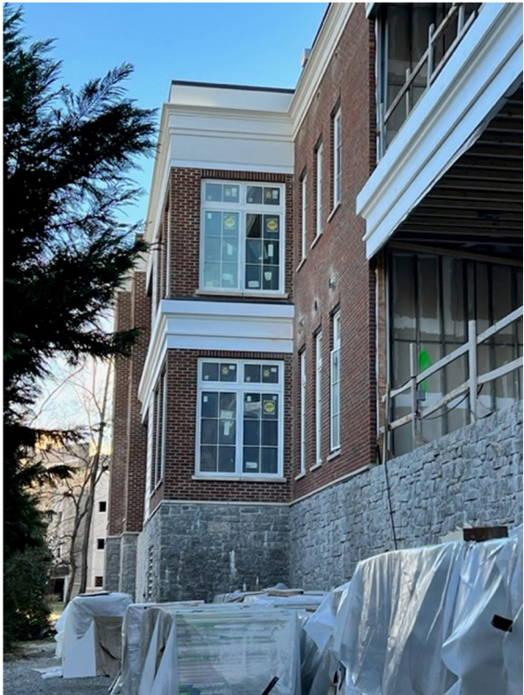
VIEW AT EXISTING SUN PORCH
