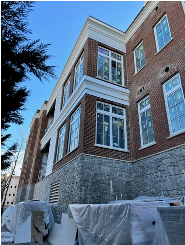
VIEW AT EXISTING SUN PORCH
