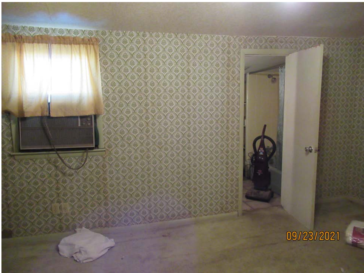
Photograph 62: Overview of right rear room at second floor.
