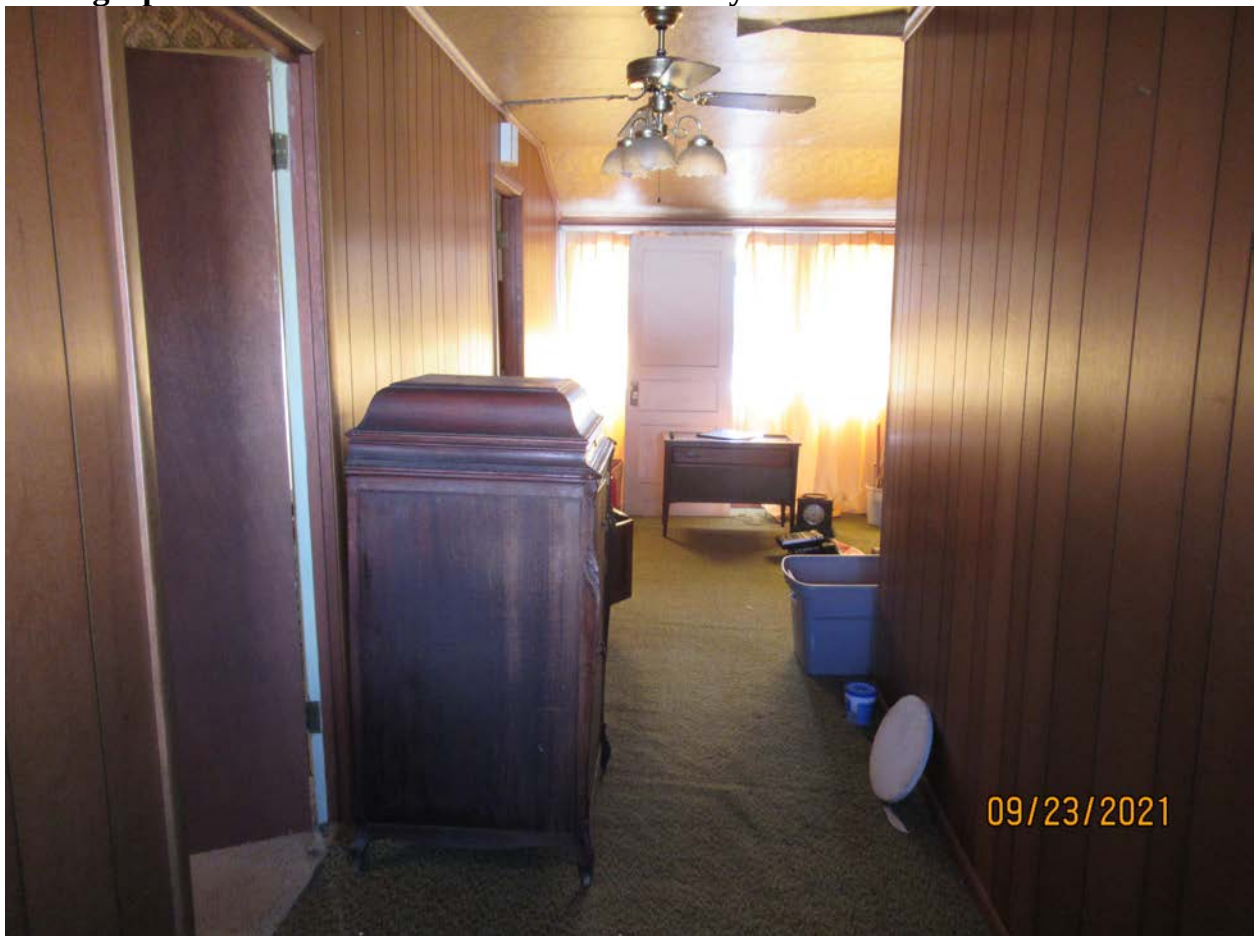
Photograph 57: Overview of second floor hallway.
