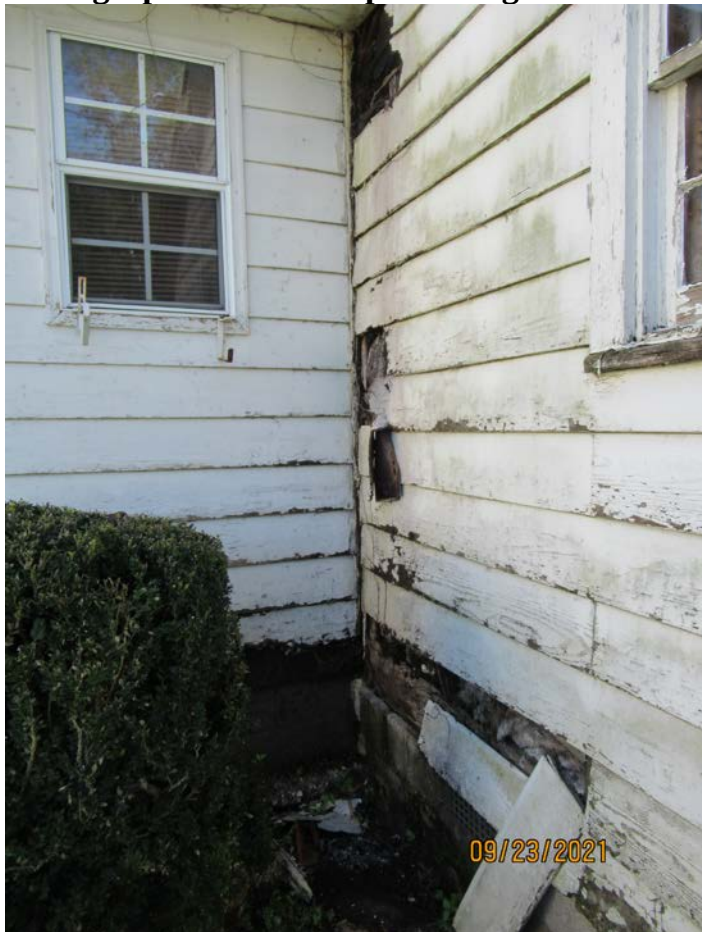
Photograph 22: Close-up of siding at kitchen area.
