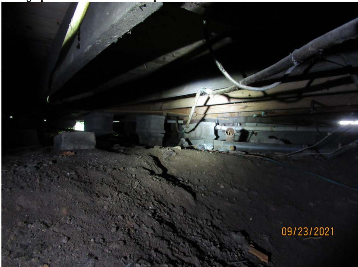
Photograph 87: Overview of crawlspace.
