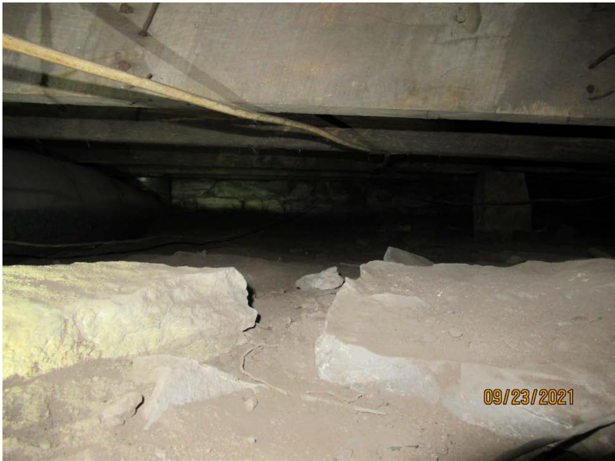
Photograph 74: Overview of crawlspace.
