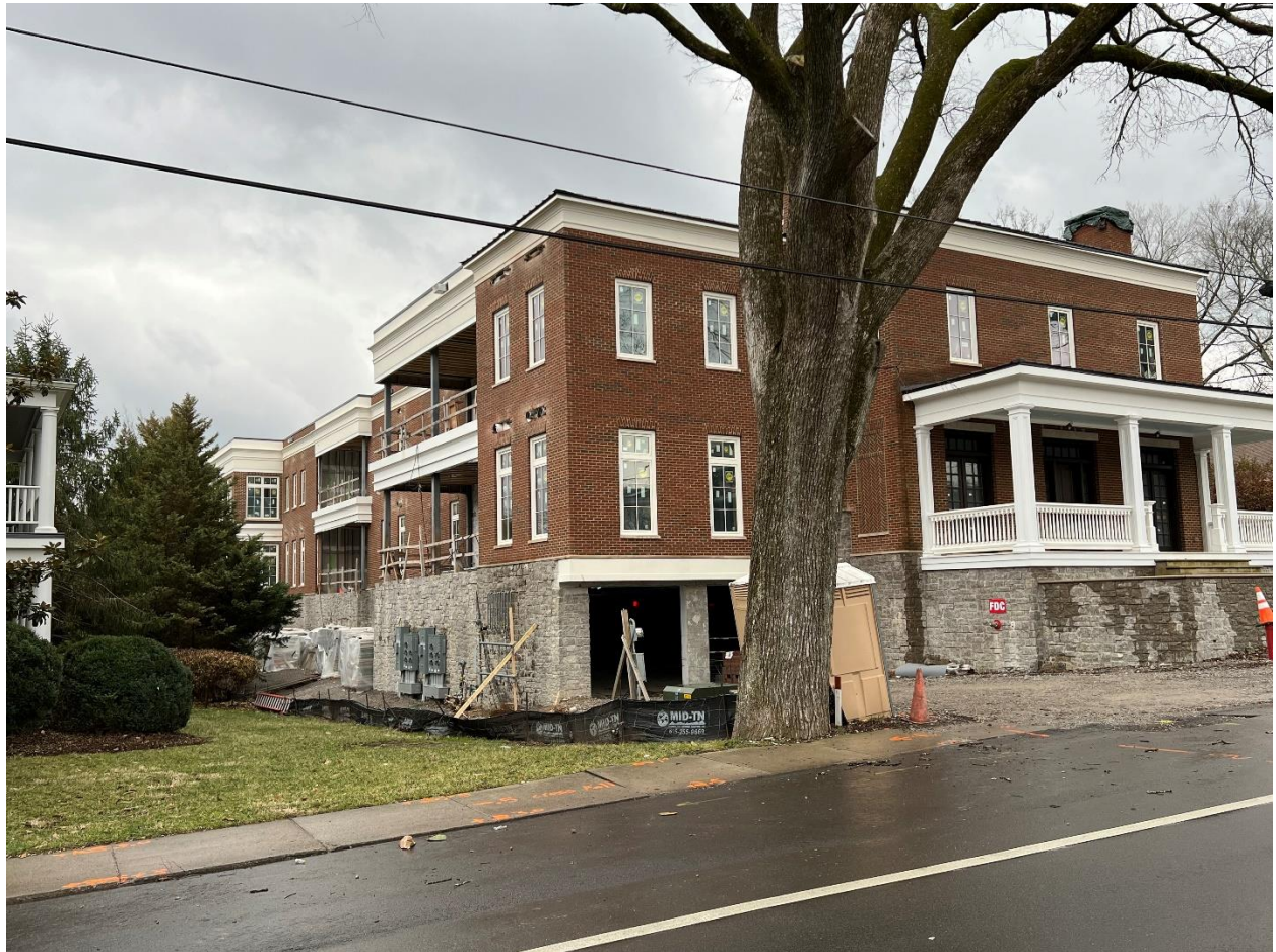
Image One: View from West Main Street toward back side of building. Note the more open porches on the front side of the building and the enclosed porches towards the rear of the lot. The face of the newly enclosed porches is approximately 250 ft back from the street to the face of the porch.
