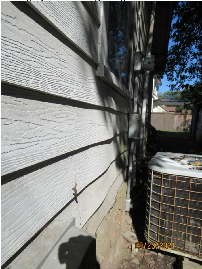
Photograph 16: Siding at right side.
