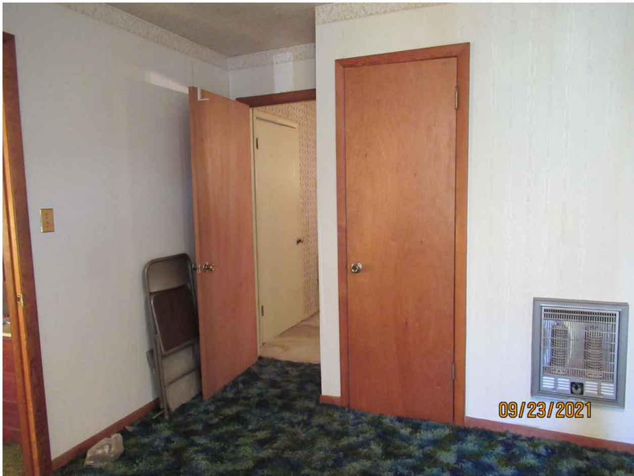
Photograph 60: Overview of right front room at second floor.
