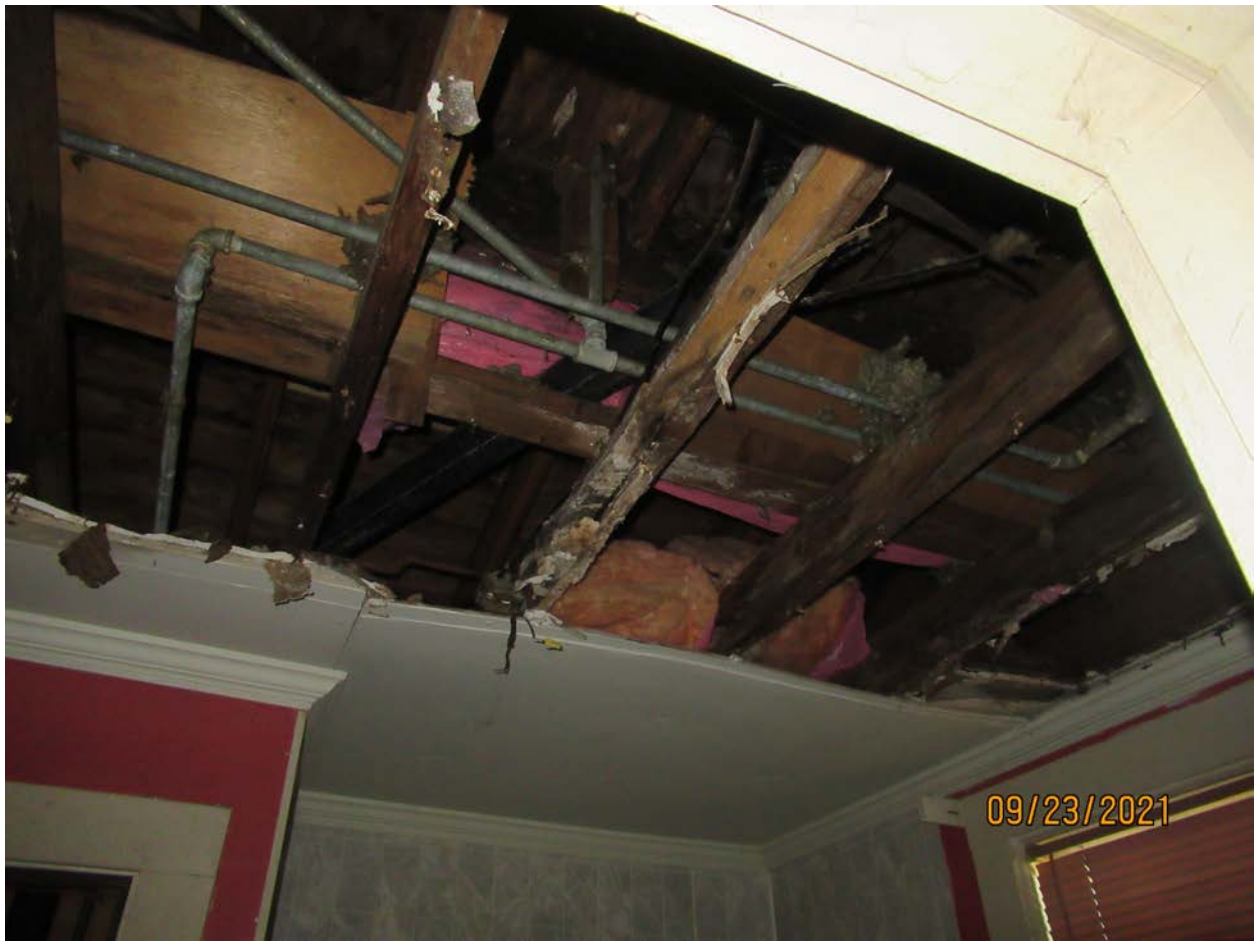
Photograph 46: First floor bathroom ceiling and floor overhead.
