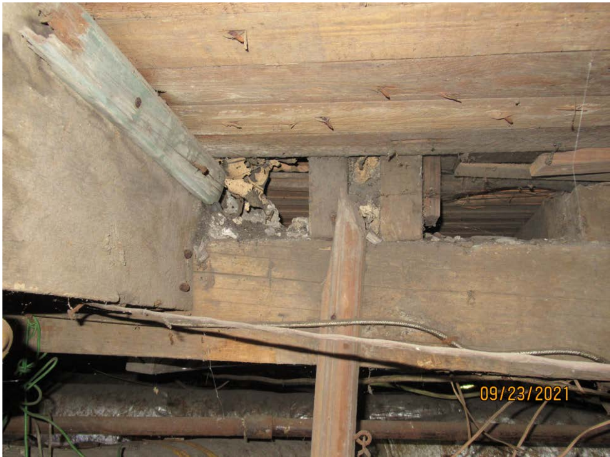
Photograph 90: Close-up of hallway wall.
