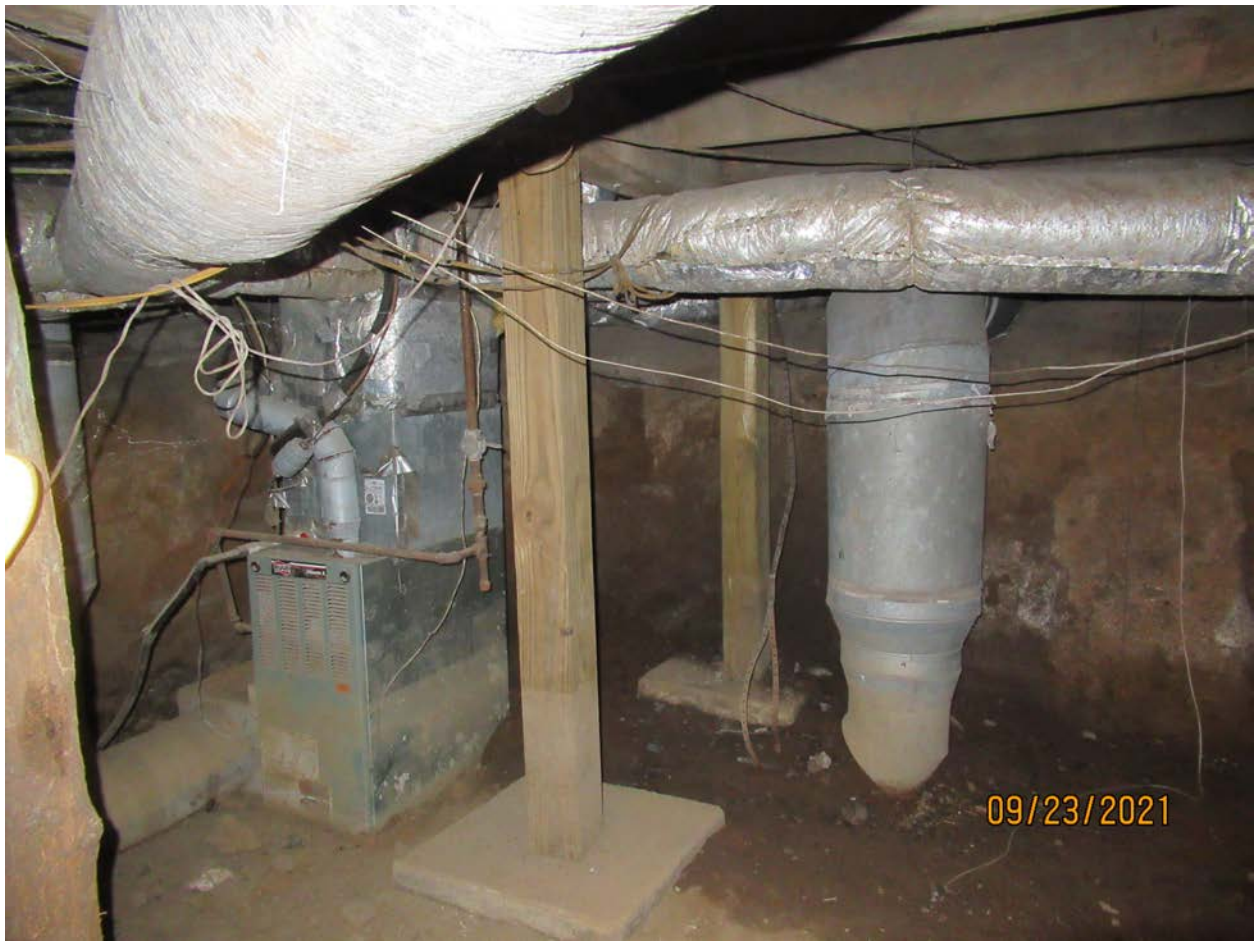
Photograph 78: Overview of cellar area.
