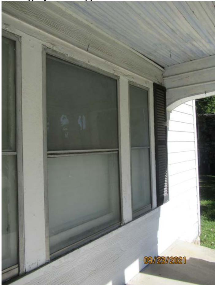
Photograph 10: Typical storm windows at front porch.
