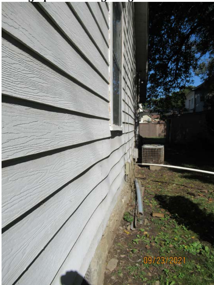
Photograph 14: Siding at right side.
