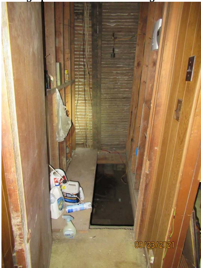
Photograph 55: Overview of ceiling access.
