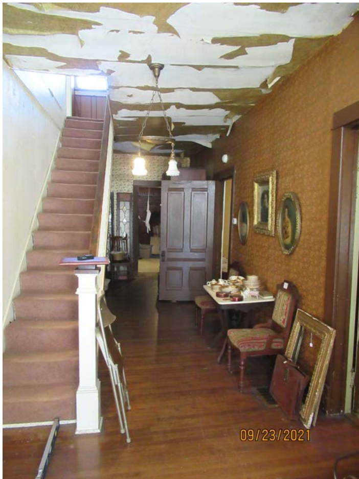
Photograph 34: Overview of hallway.
