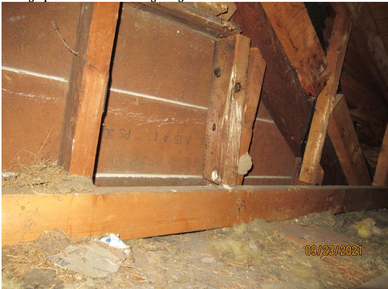
Photograph 101: Masonite siding at right-side wall.
