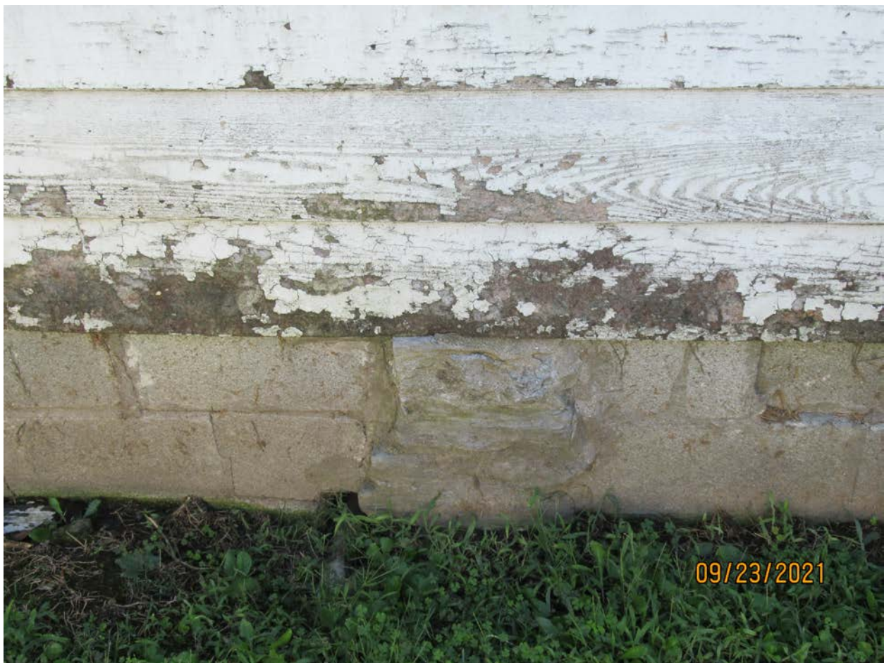
Photograph 23: Possible stone piers at rear wall addition.
