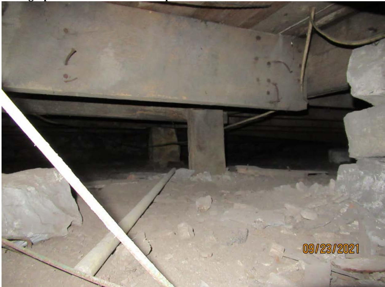
Photograph 73: Overview of crawlspace.
