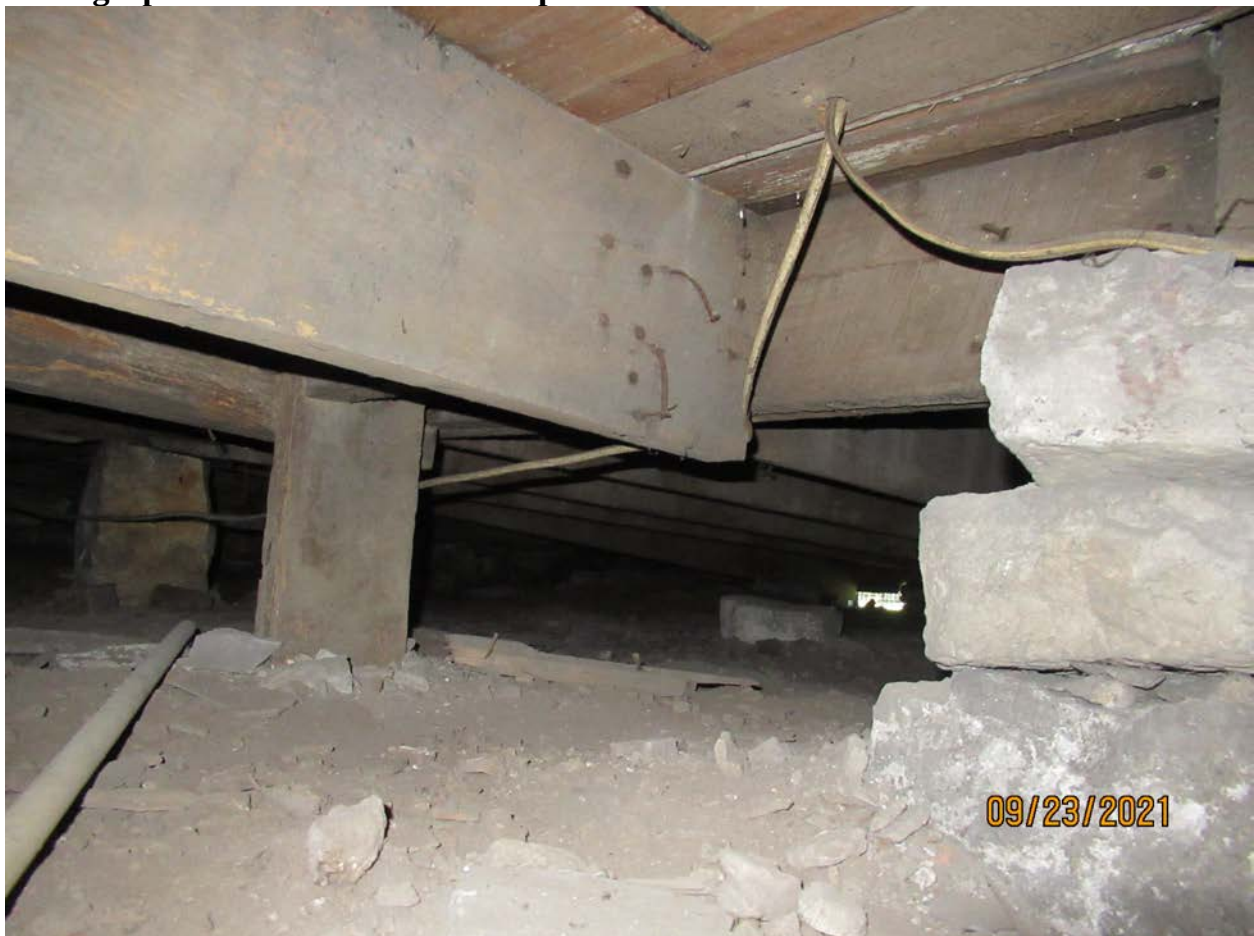
Photograph 77: Overview of crawlspace.
