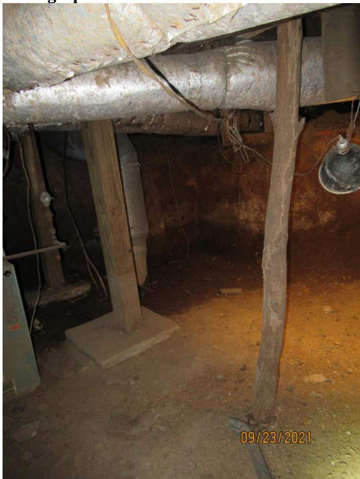
Photograph 79: Overview of cellar area.
