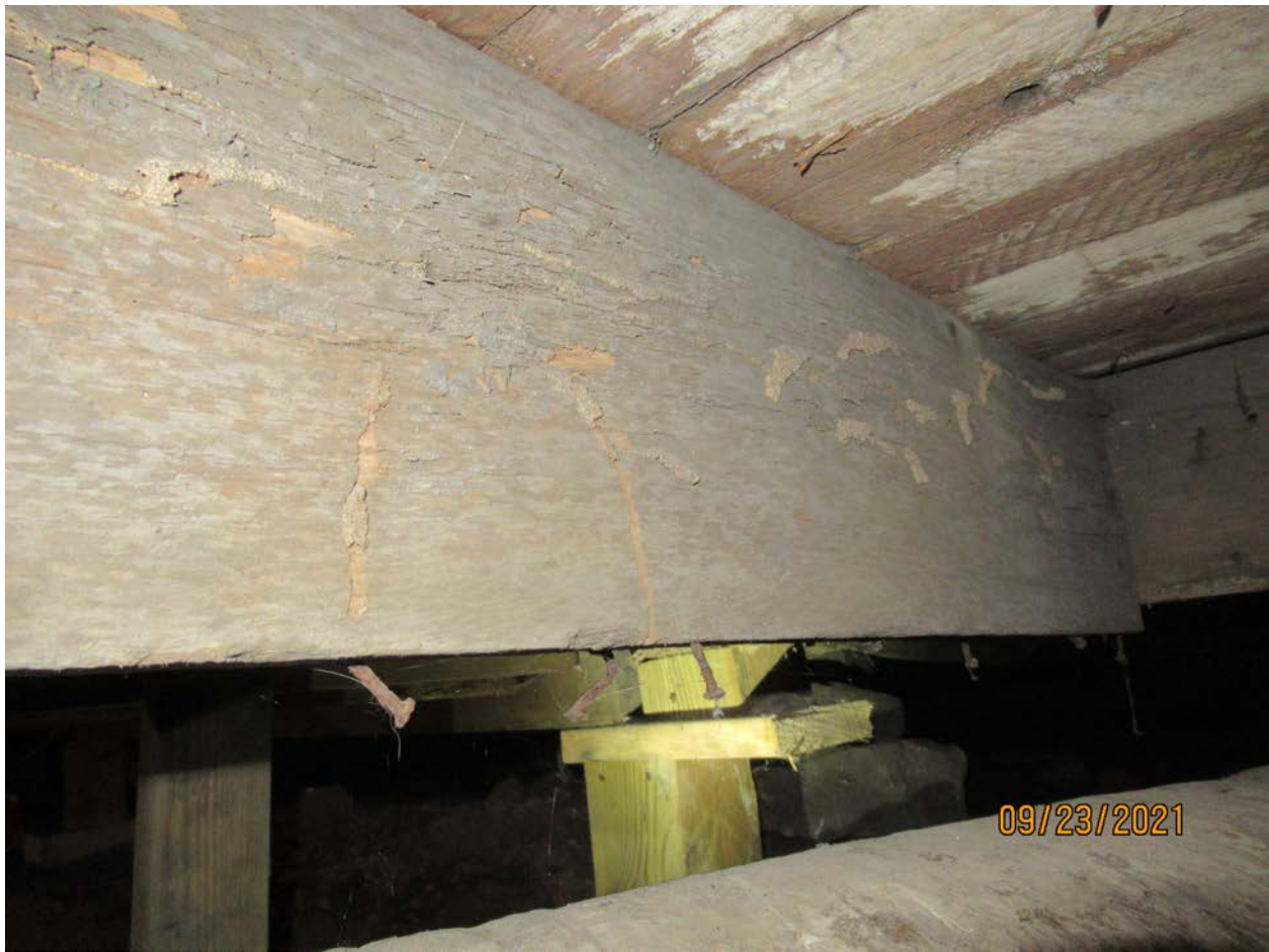
Photograph 88: Overview of crawlspace.
