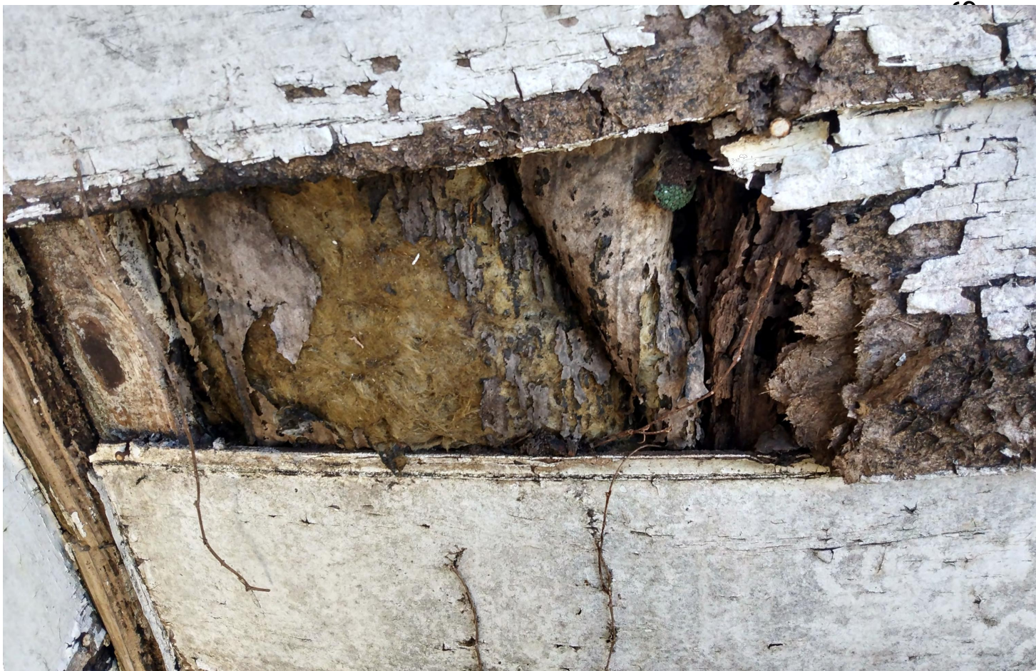
EXPOSED INSULATION
