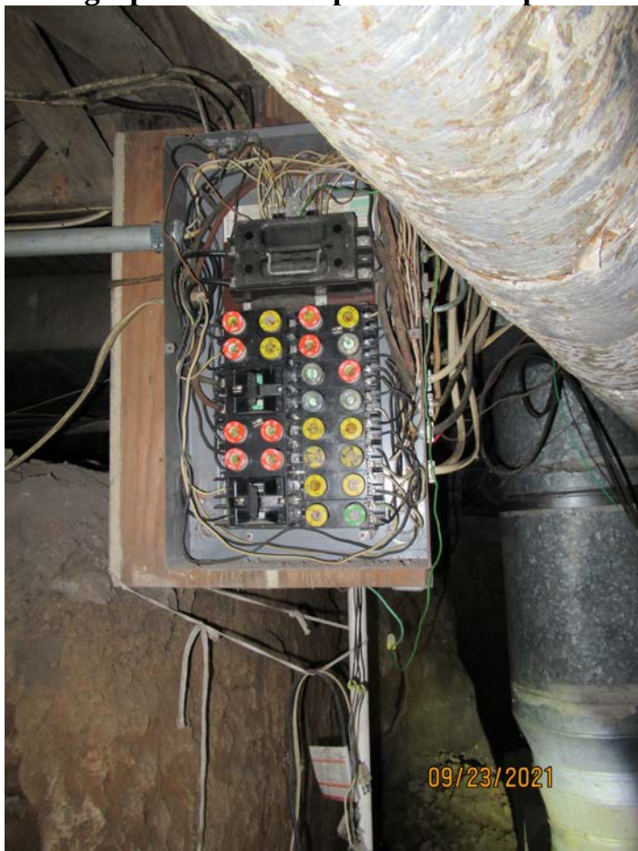
Photograph 85: Close-up of electrical panel.
