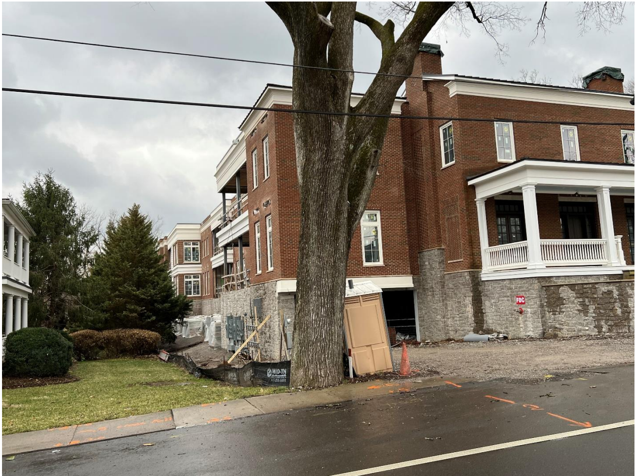
Image No. 2: View of infilled porch from West Main Street.
