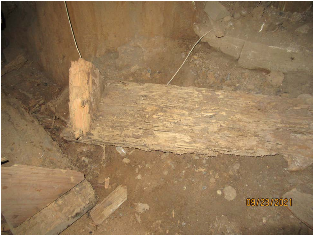
Photograph 98: Close-up of stairs to cellar.
