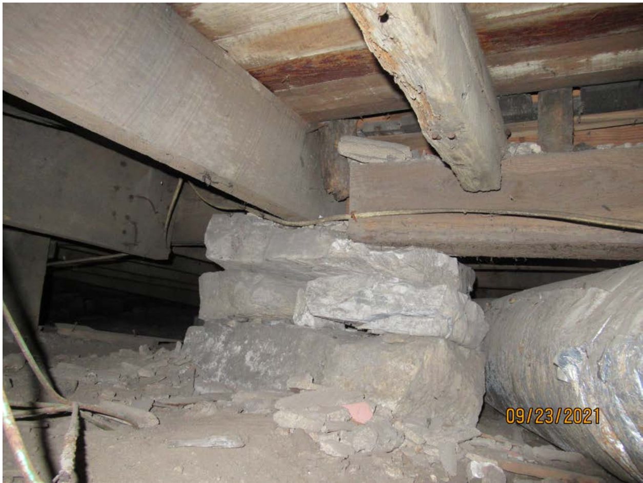
Photograph 72: Overview of crawlspace.
