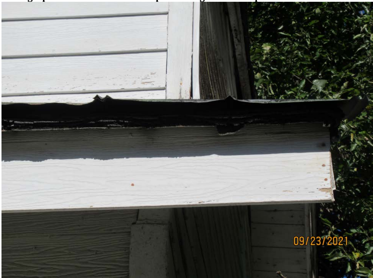
Photograph 12: Metal roof over asphalt shingles at front porch.
