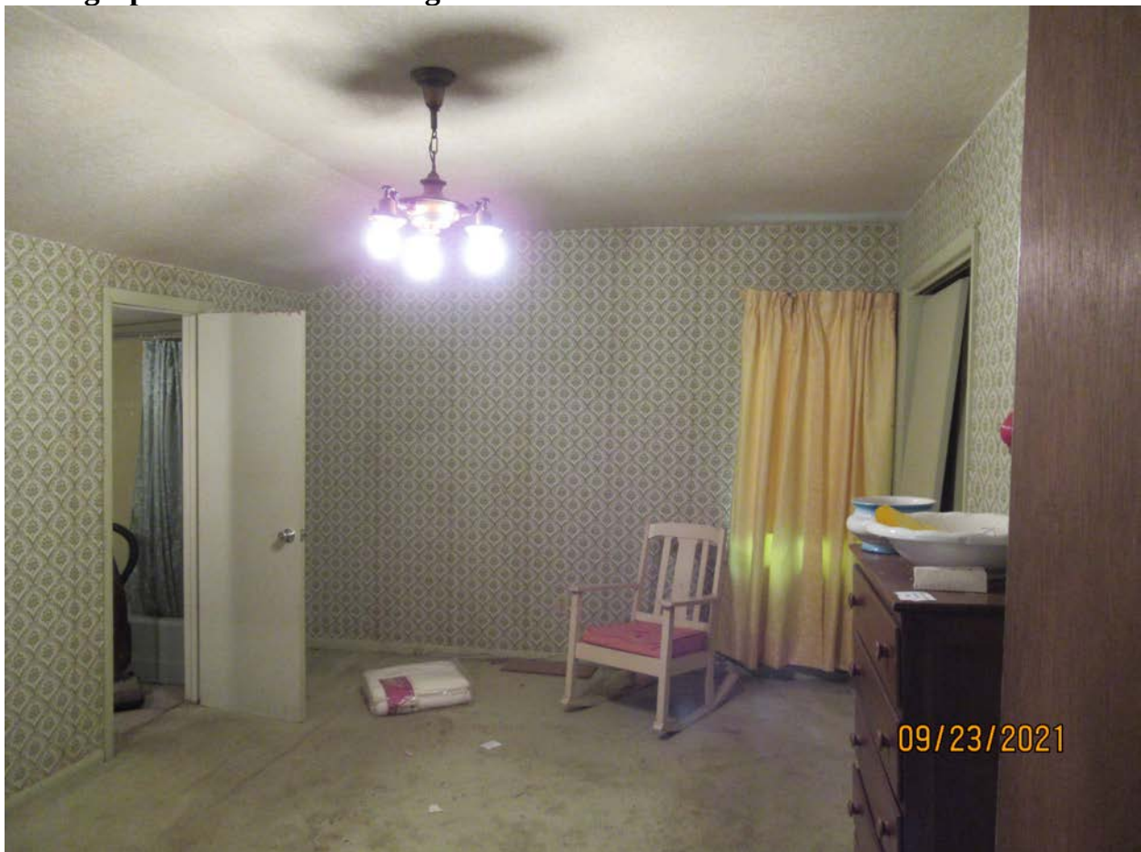
Photograph 61: Overview of right rear room at second floor.
