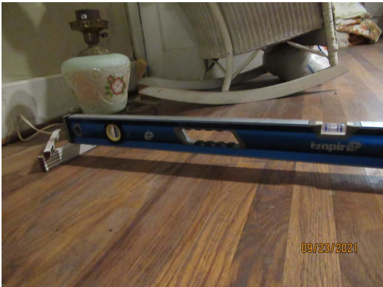
Photograph 42: Overview of flat floor at right rear room at main floor.
