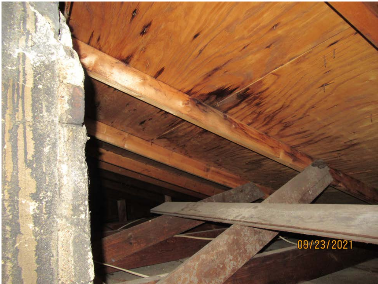
Photograph 100: Overview of attic framing.
