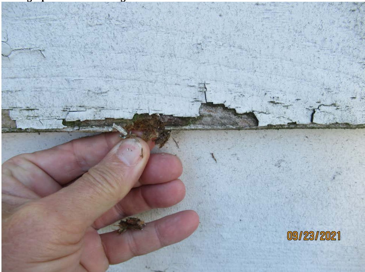
Photograph 20: Fiber siding at rear elevation.
