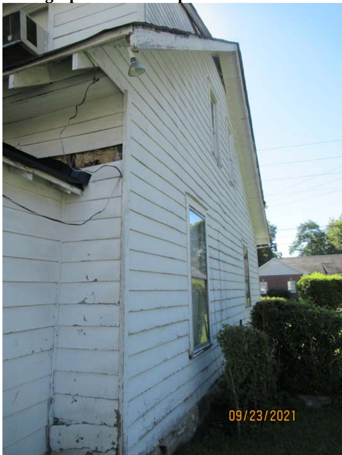
Photograph 28: Close-up of left-side wall at addition.
