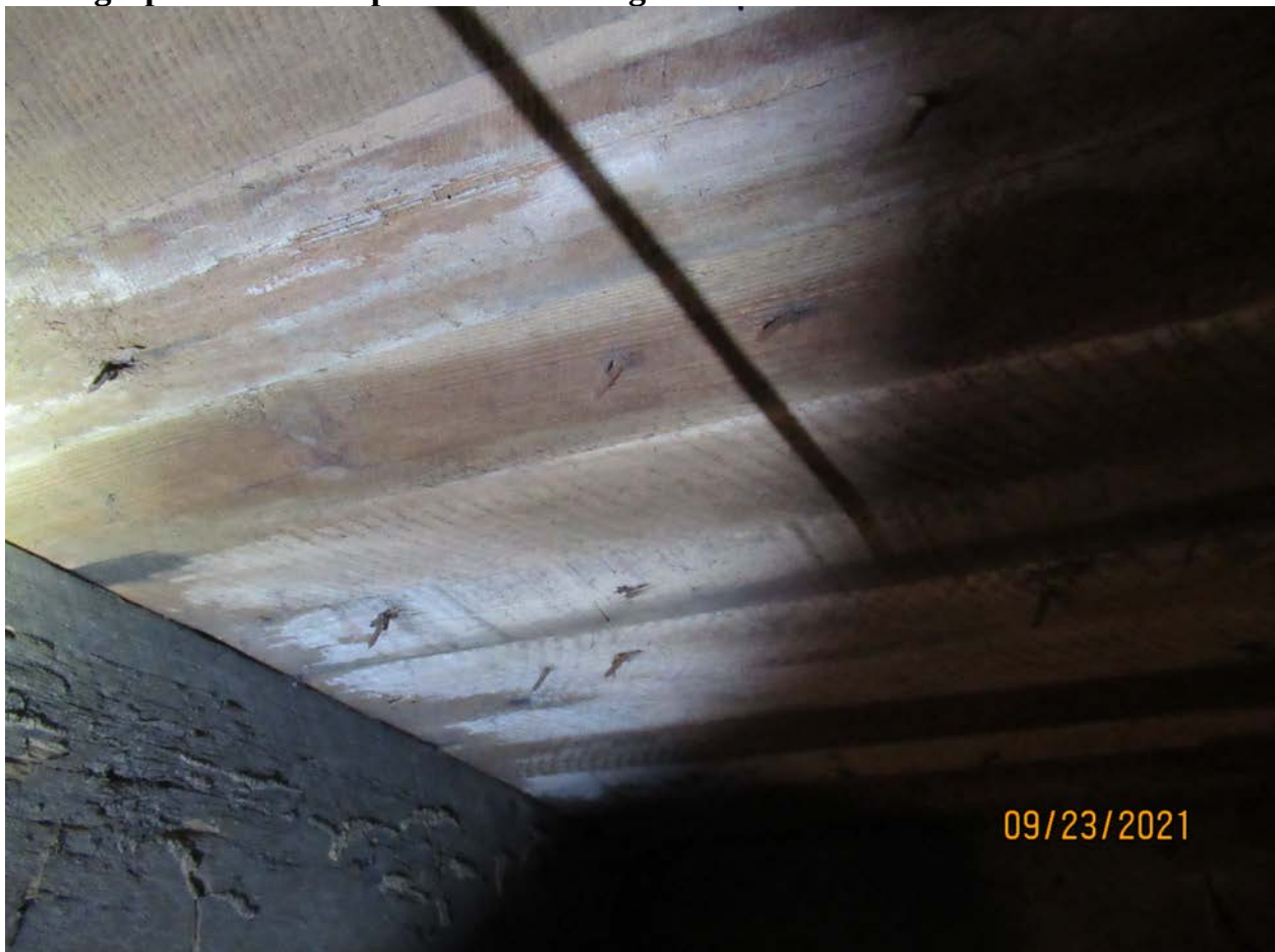
Photograph 89: Close-up of wood flooring.
