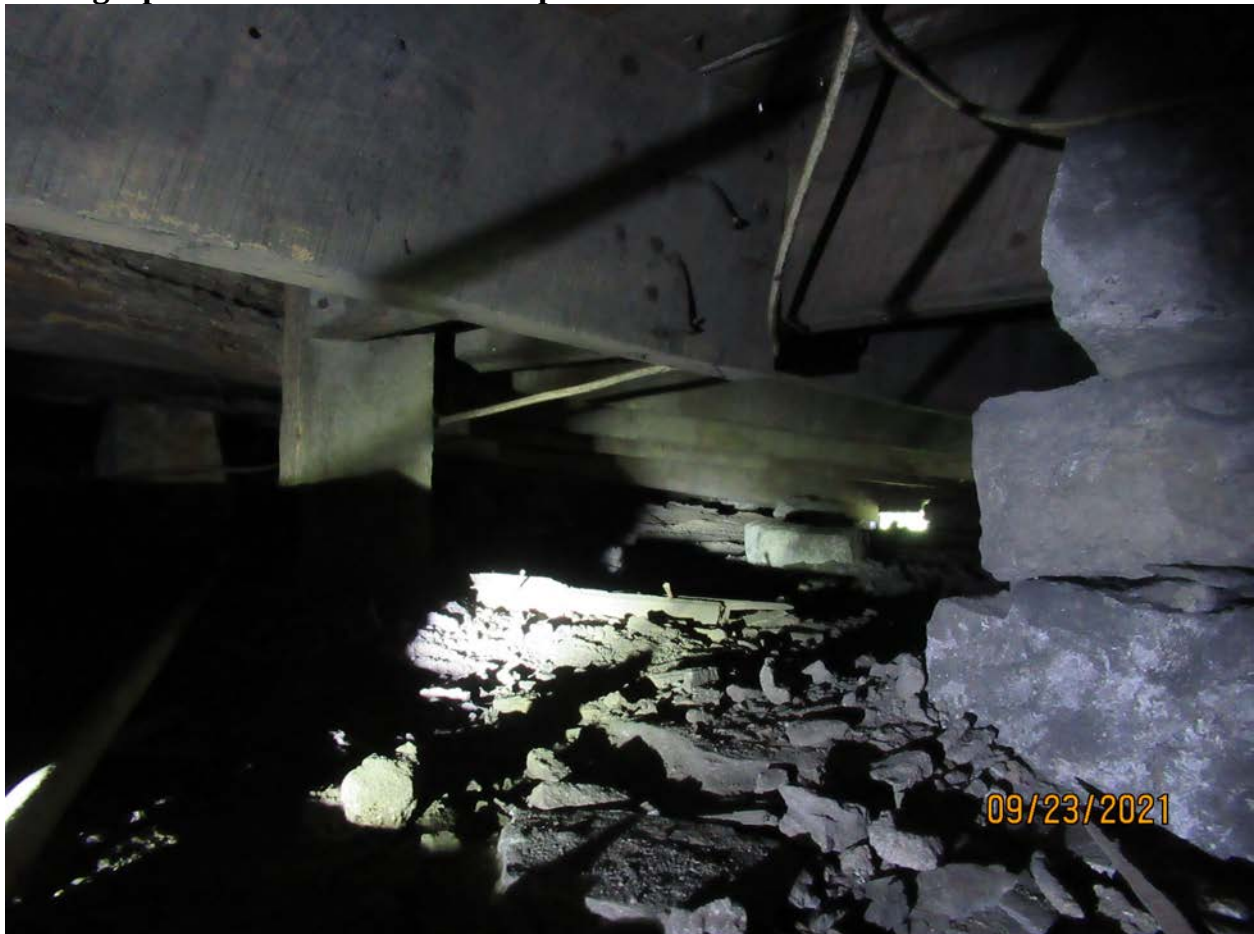
Photograph 75: Overview of crawlspace.
