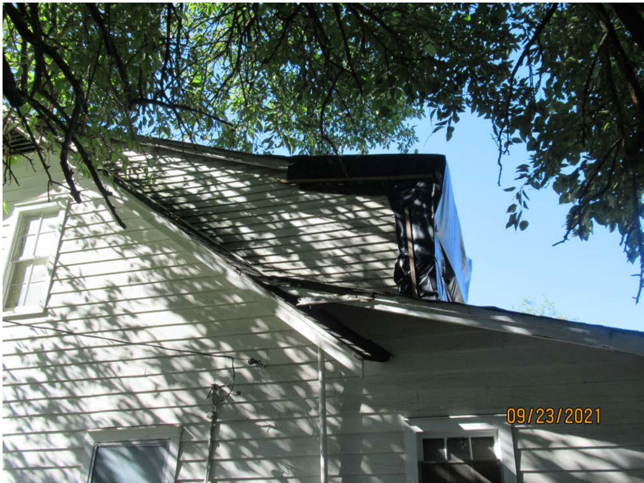
Photograph 17: Right-side elevation at second floor restroom.
