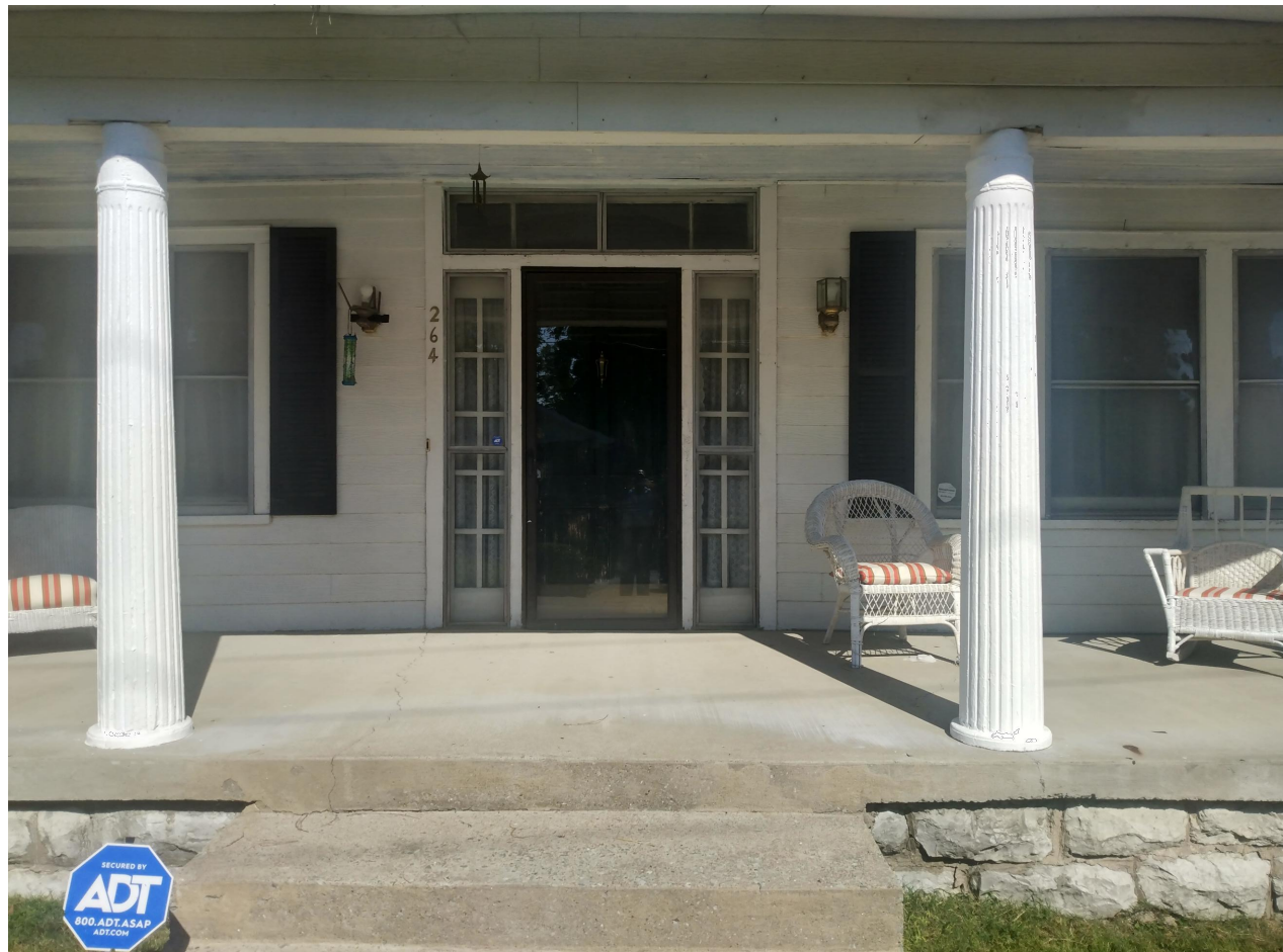
MAIN ENTRANCE - FRONT
