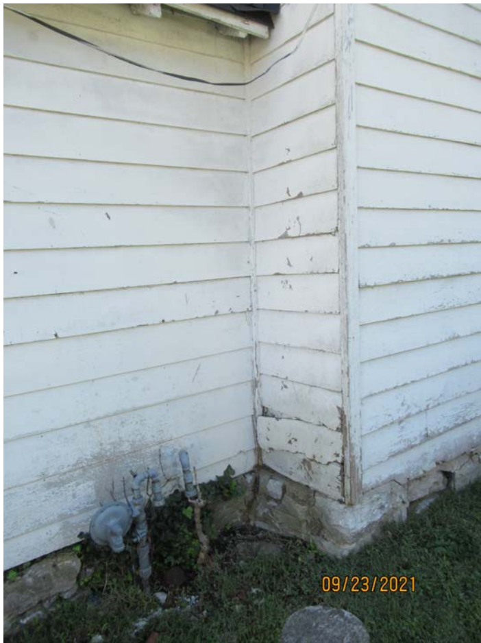
Photograph 27: Close-up of left-side wall at addition.
