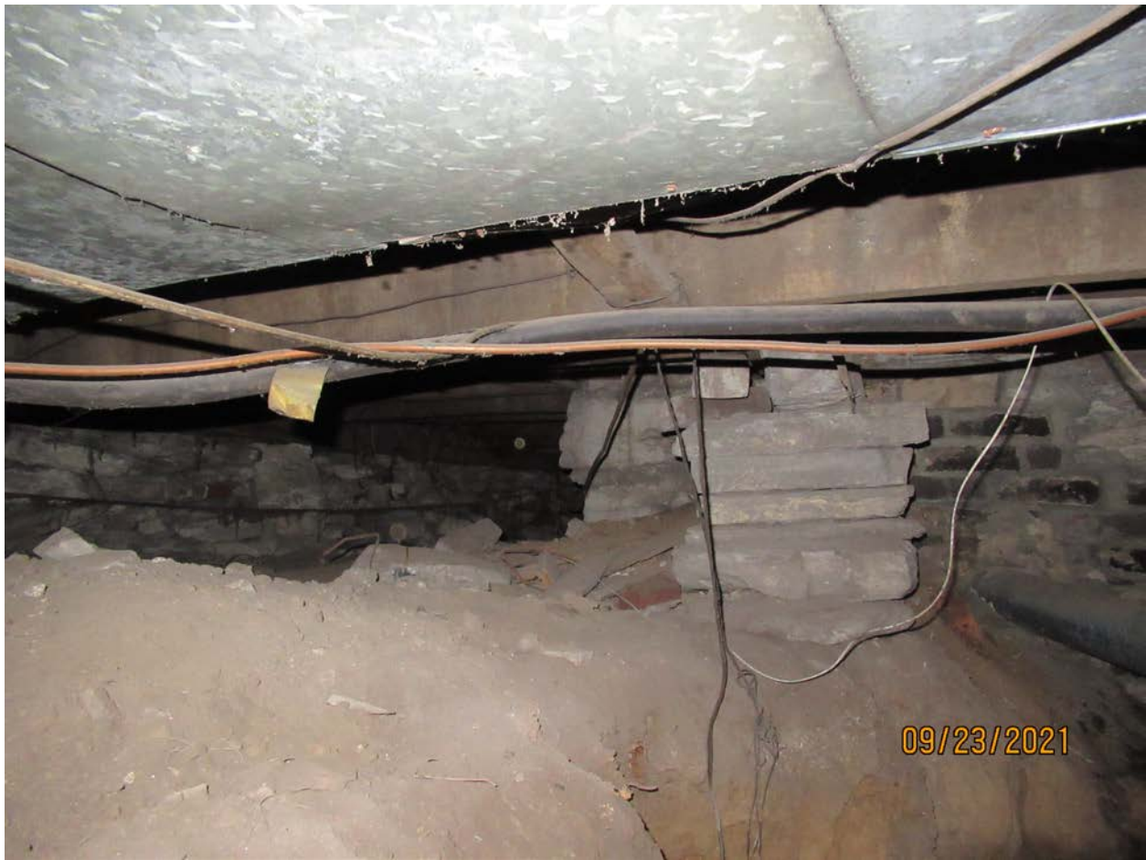
Photograph 80: Overview of crawlspace.
