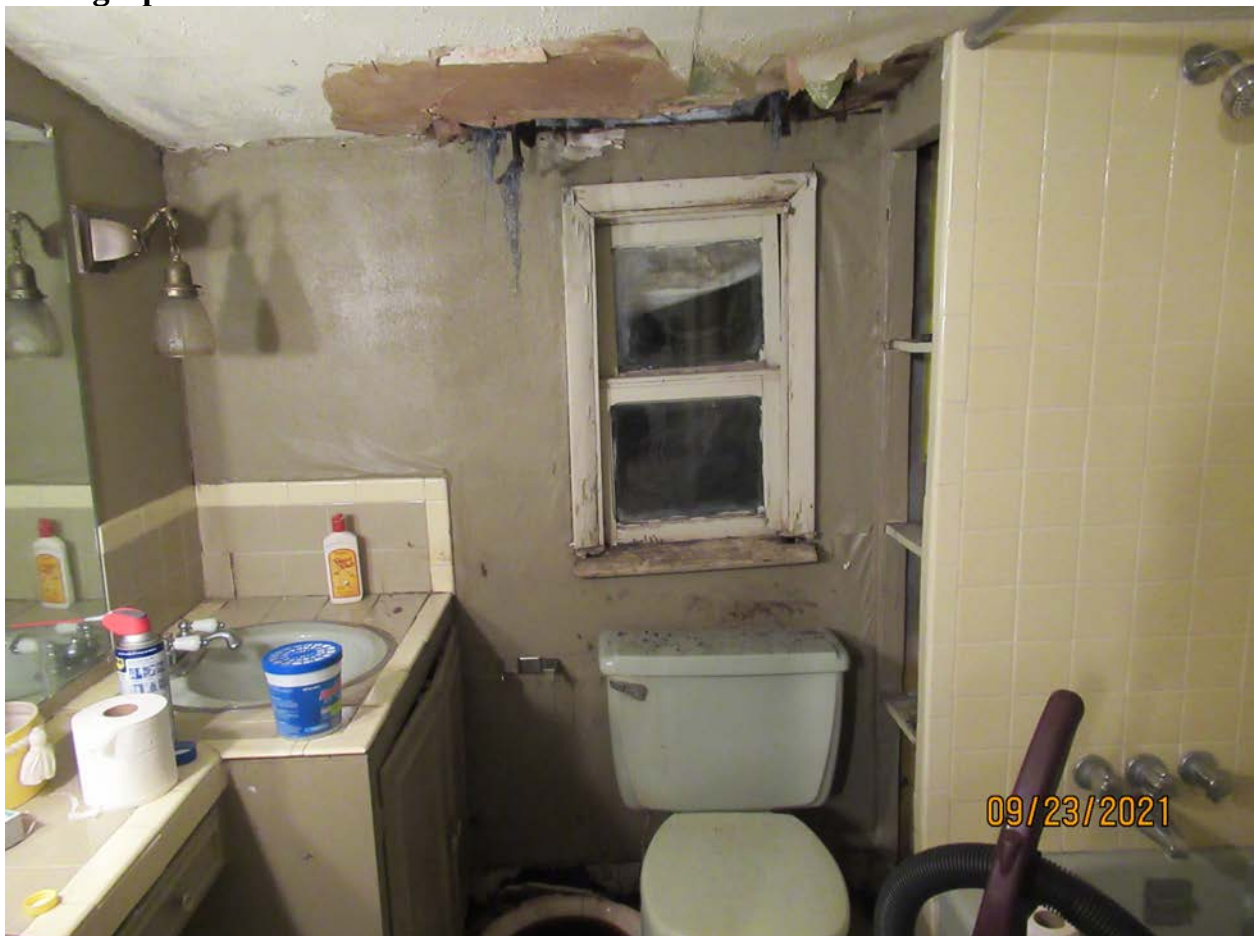
Photograph 63: Overview of second floor bathroom.
