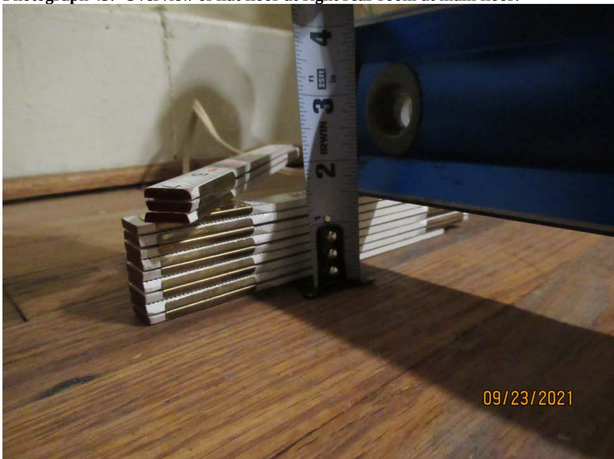
Photograph 43: Overview of flat floor at right rear room at main floor.
