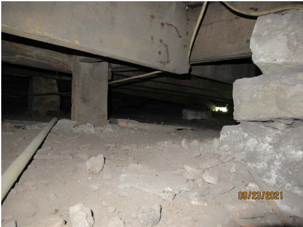
Photograph 76: Overview of crawlspace.
