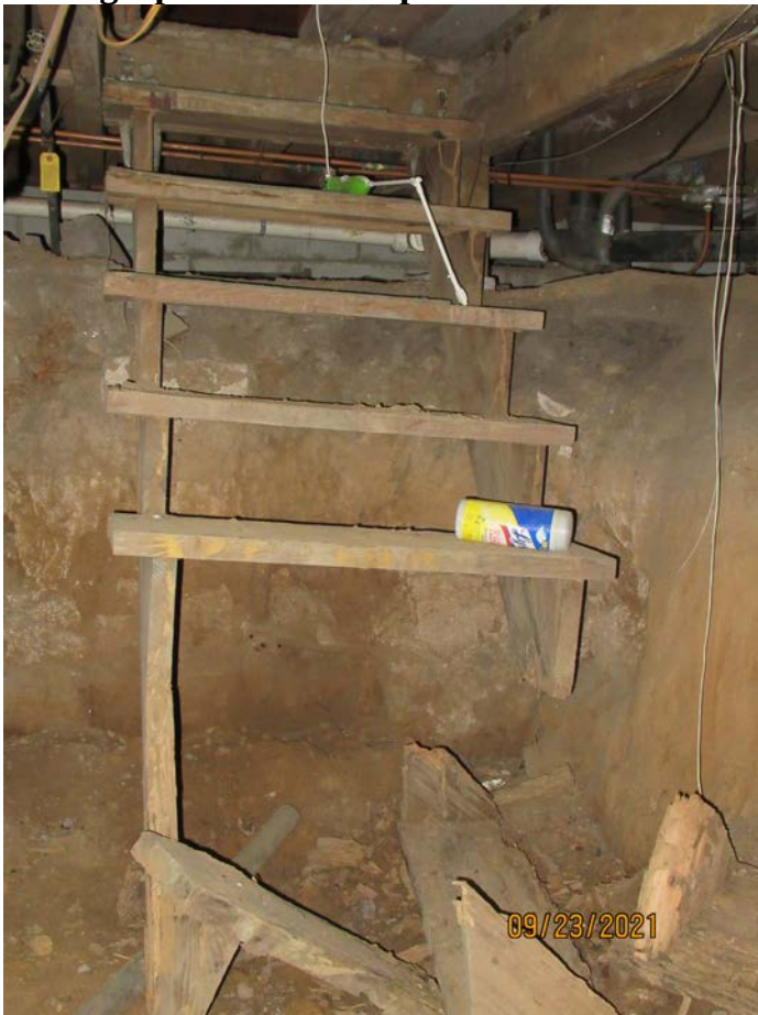
Photograph 97: Close-up of stairs to cellar.
