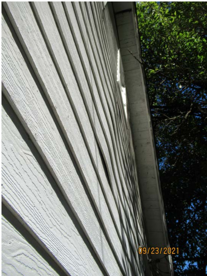
Photograph 15: Siding at right side.
