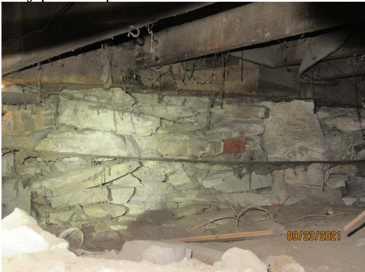
Photograph 81: Close-up of foundation wall.
