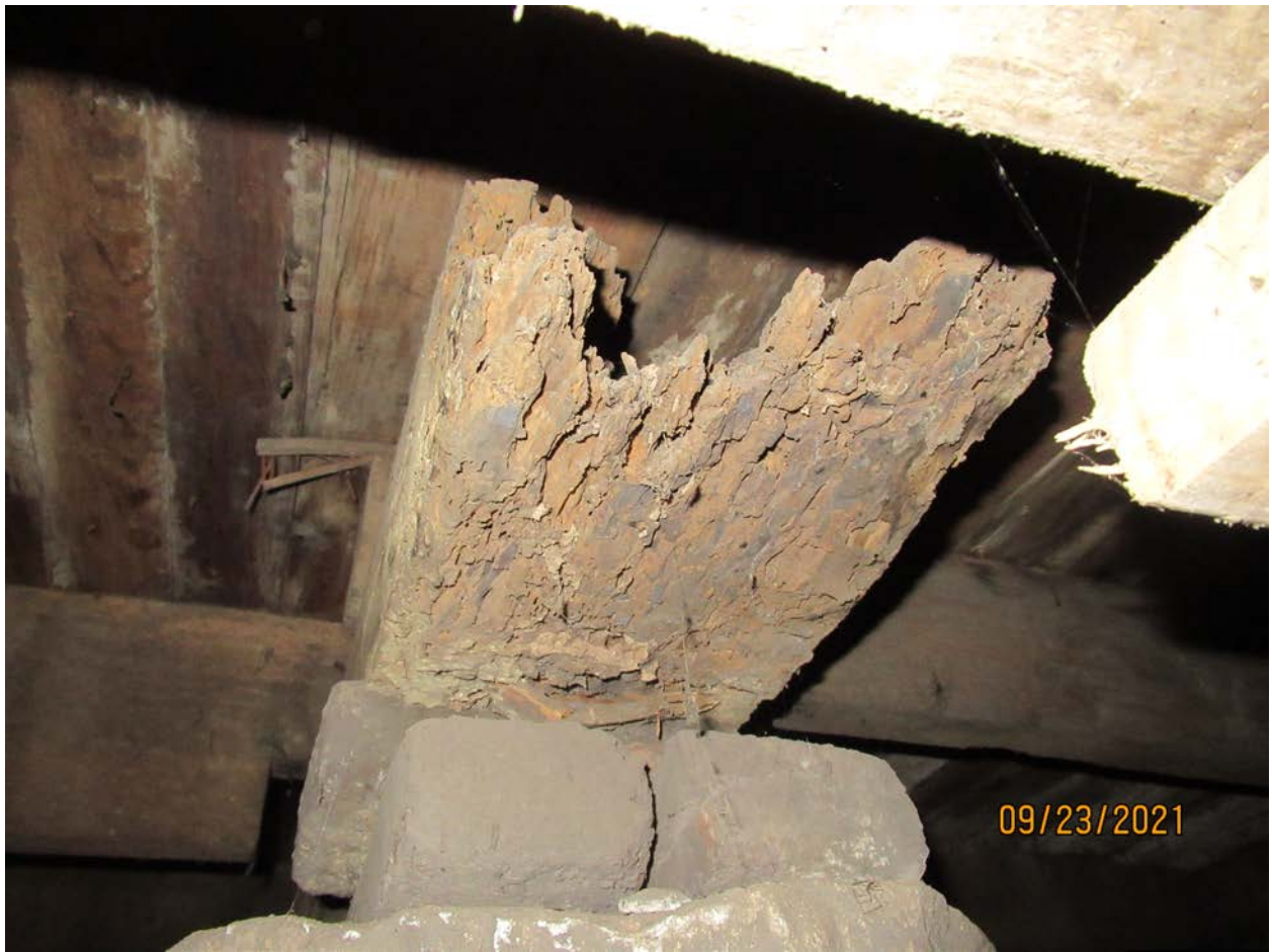
Photograph 94: Close-up of support beam at main floor.
