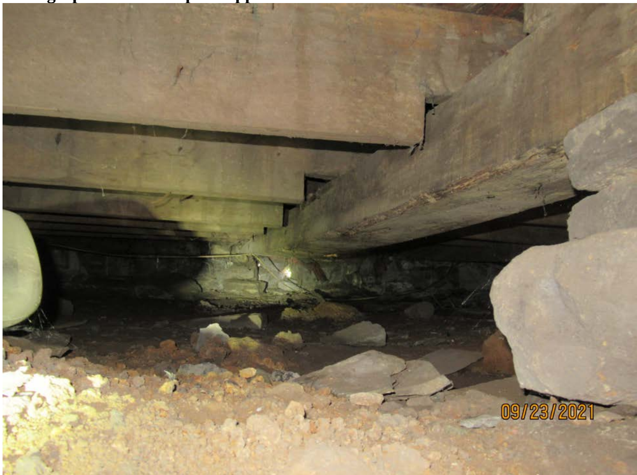
Photograph 91: Close-up of support beam at main floor.
