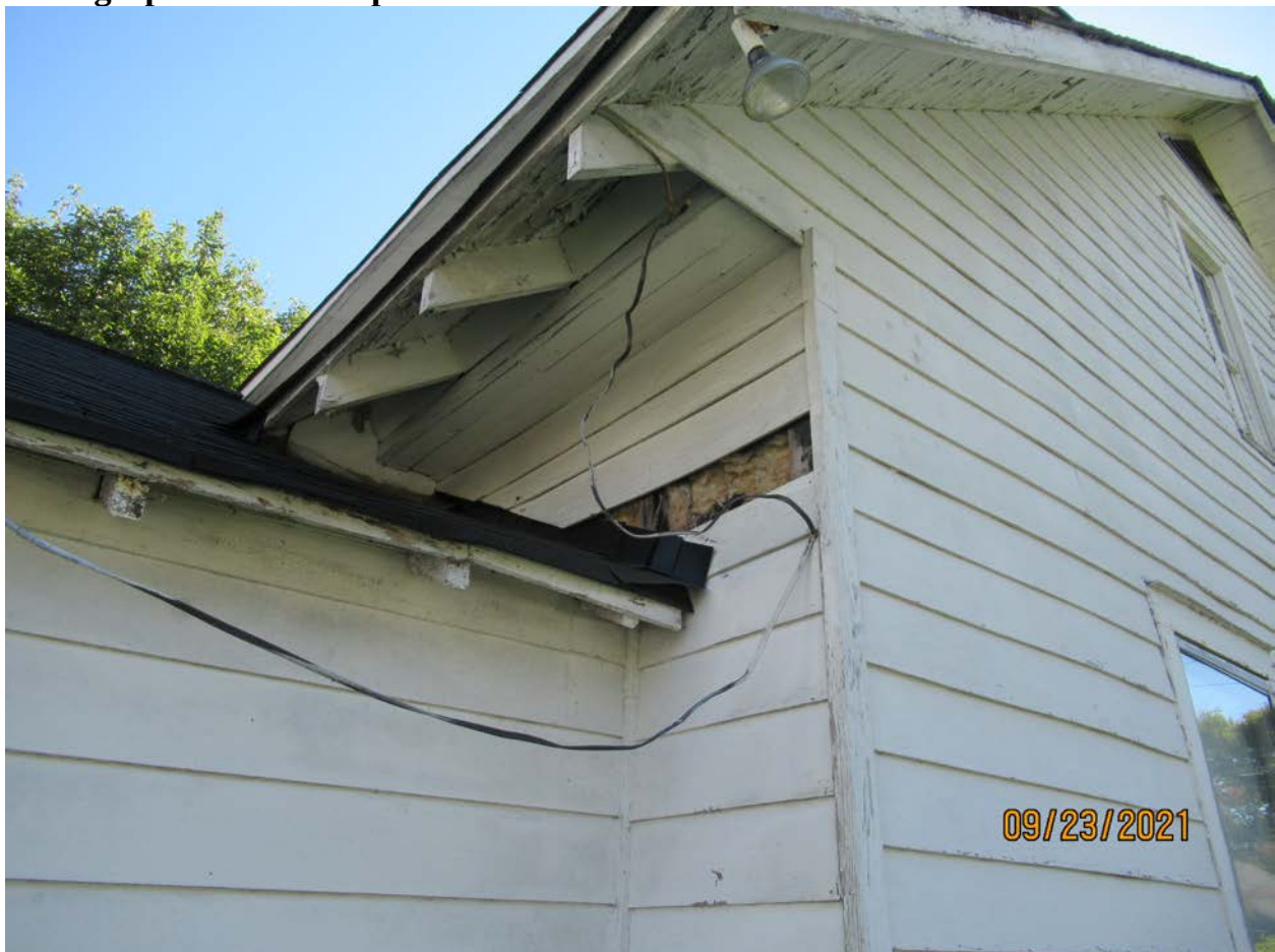
Photograph 26: Close-up of left-side wall at addition.
