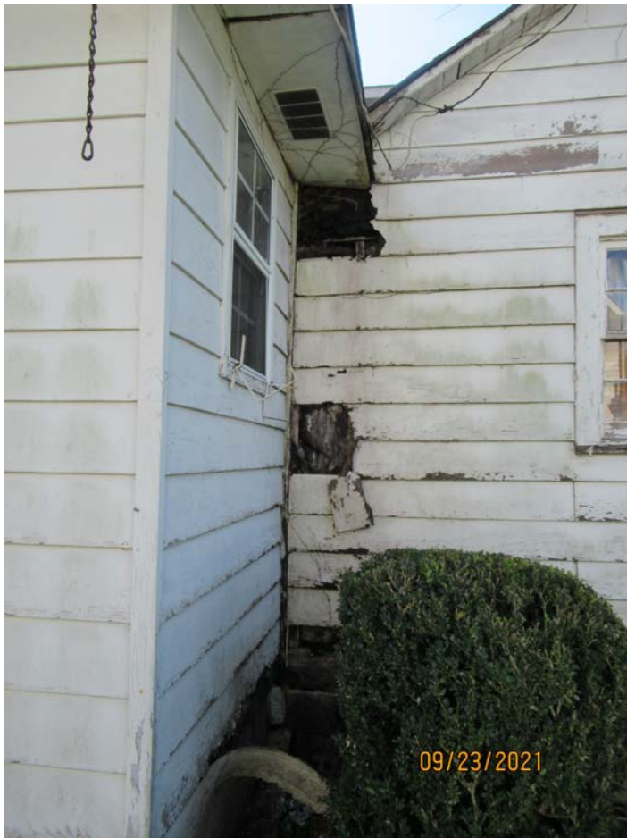
Photograph 21: Close-up of siding at kitchen area.
