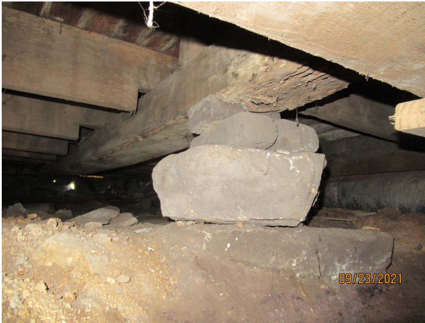
Photograph 93: Close-up of support beam at main floor.
