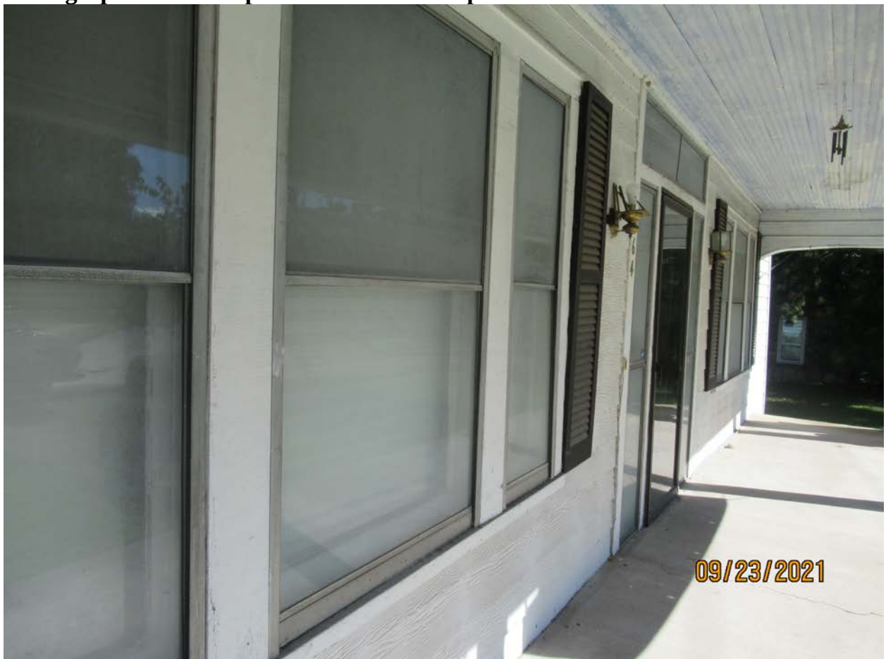
Photograph 4: Close-up of front wall below porch roof.
