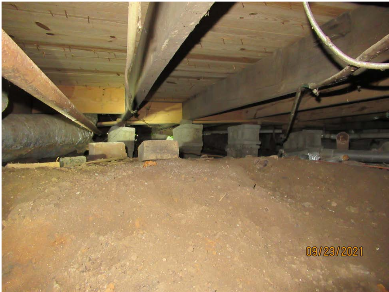
Photograph 86: Overview of crawlspace.
