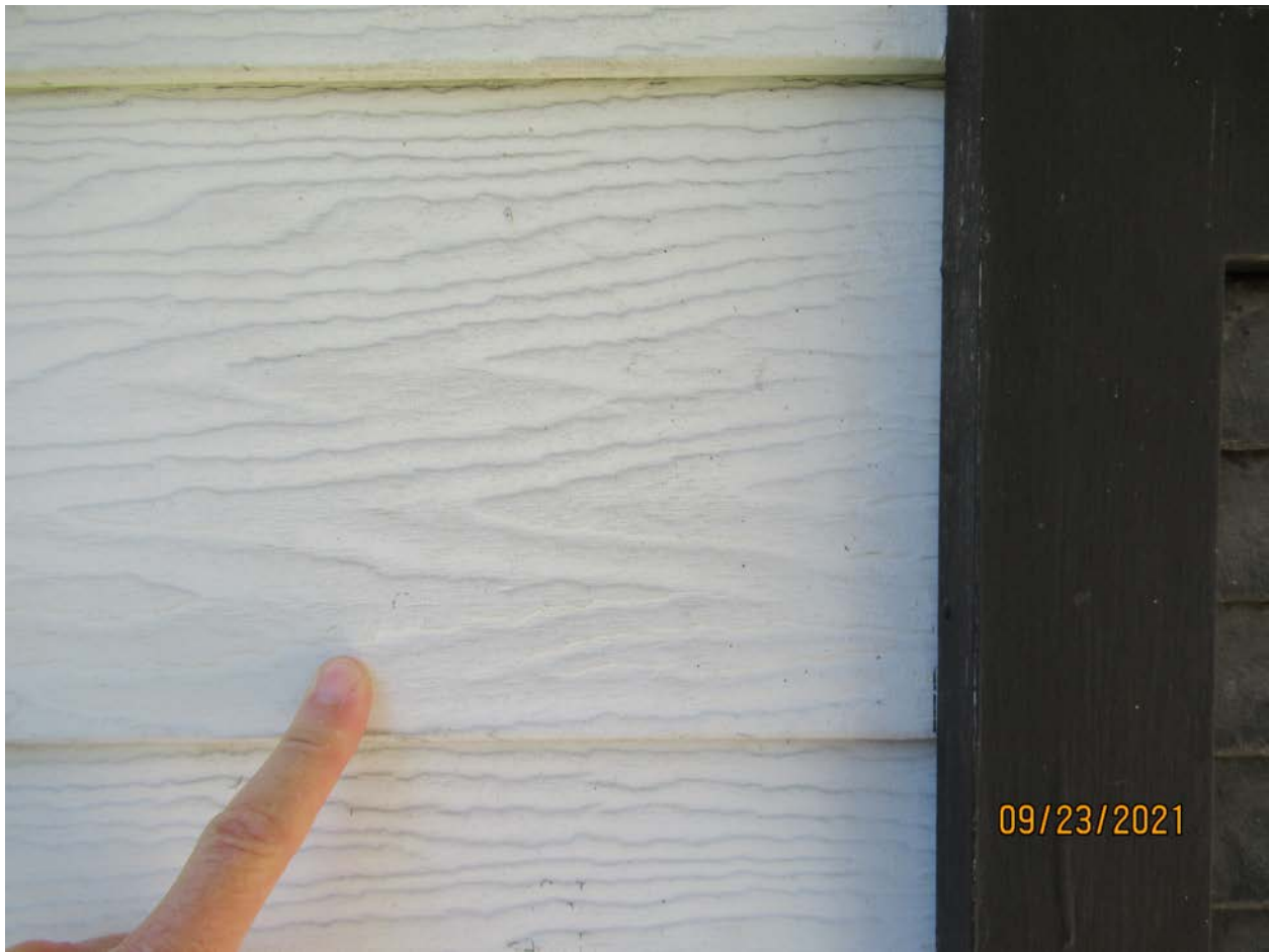
Photograph 5: Typical siding at front wall.
