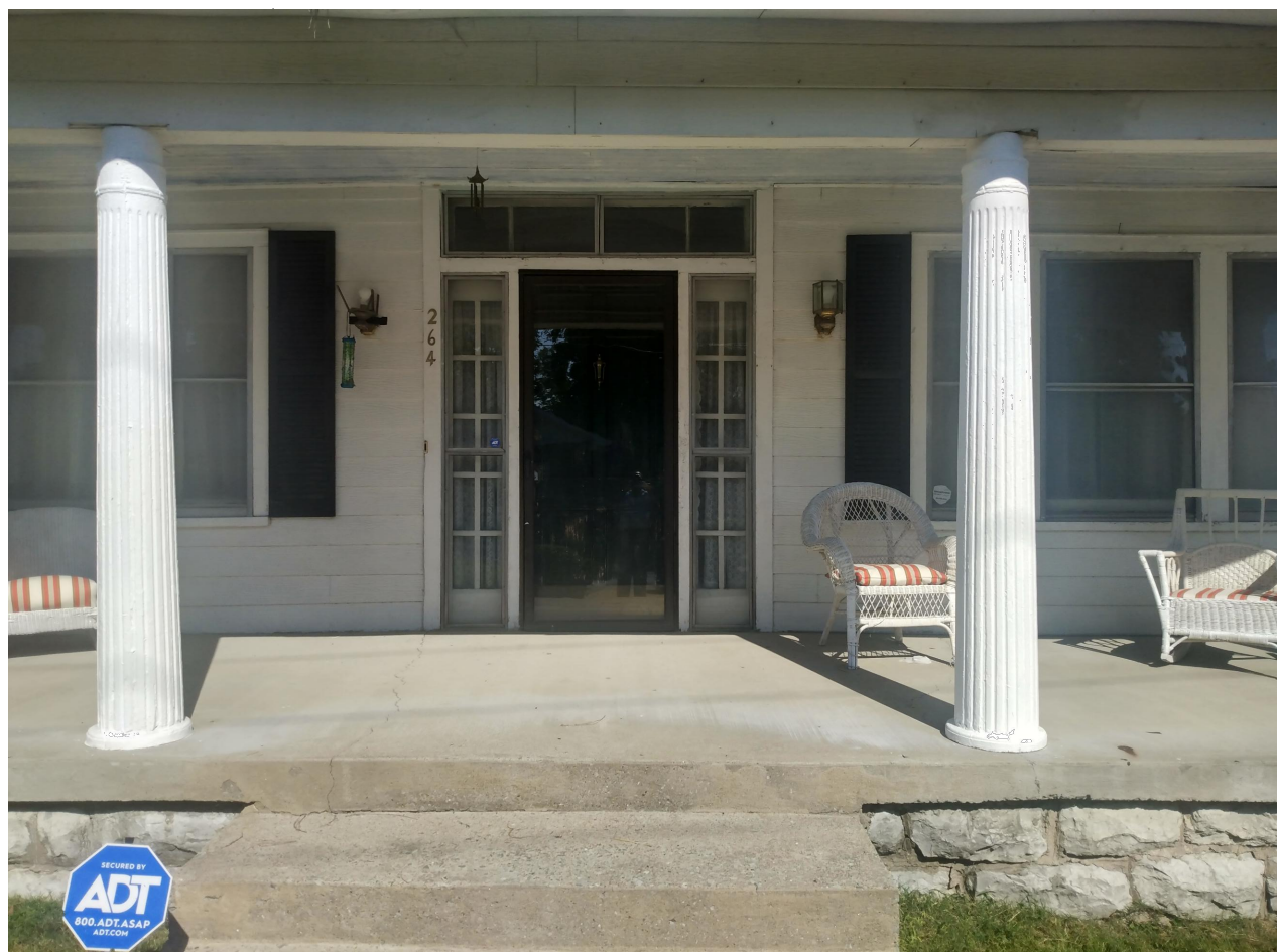
MAIN ENTRANCE - FRONT
