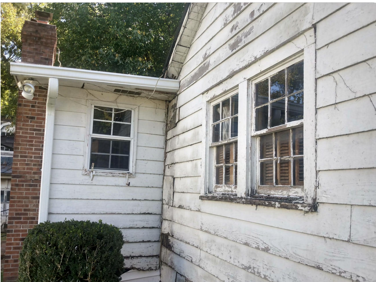
DETERIORATED SIDING
