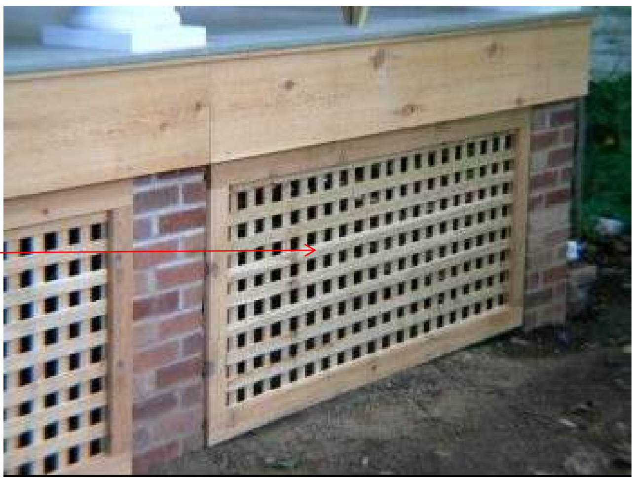
EXAMPLE OF CUSTOM SITE-FABRICATED LATTICE
