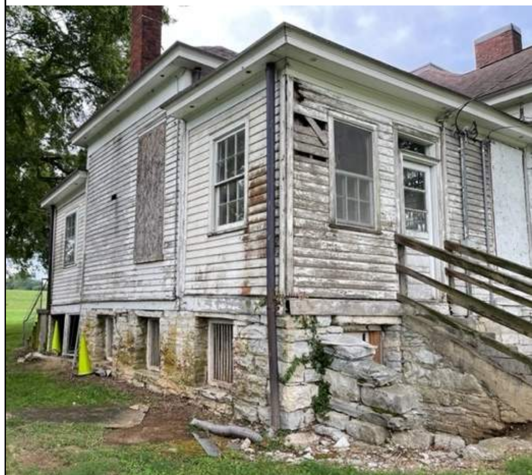
VIEW OF REAR FROM NW CORNER
