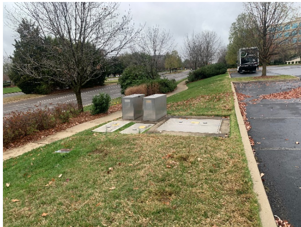
Existing utility water backflow system along subject front parking curb alignment (Looking Northwest towards Carothers from proposed building)
