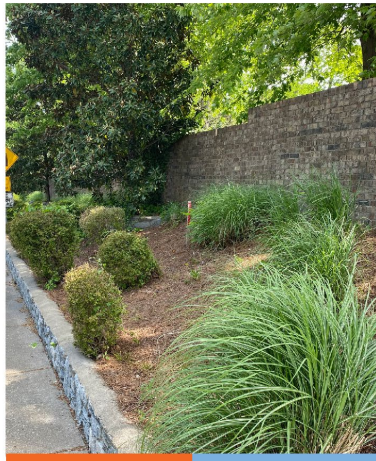
STONE & BRICK WALLS
