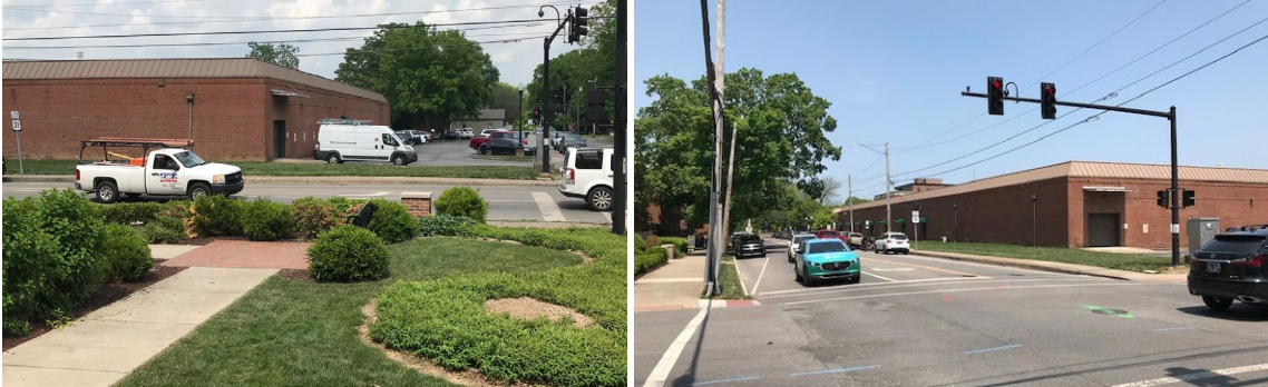
Figure 3: View of south side of city hall looking east (above left), View of city hall looking north from Church Street (above right)
