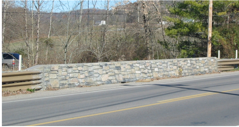
Bridge Rail Barrier
