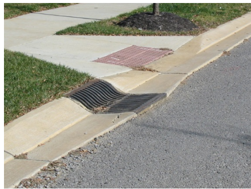
Rollover curb with grate transition
