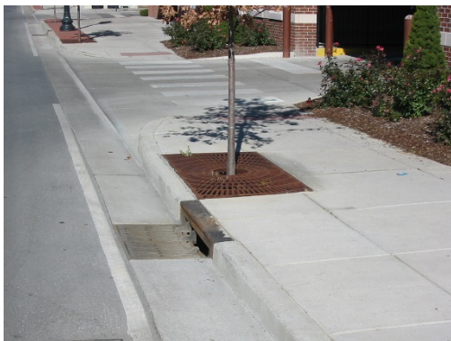
Vertical combined curb and gutter
