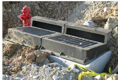
Vane grate for curb and gutter section
