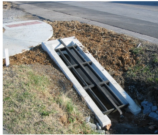
TDOT Safety Endwall
