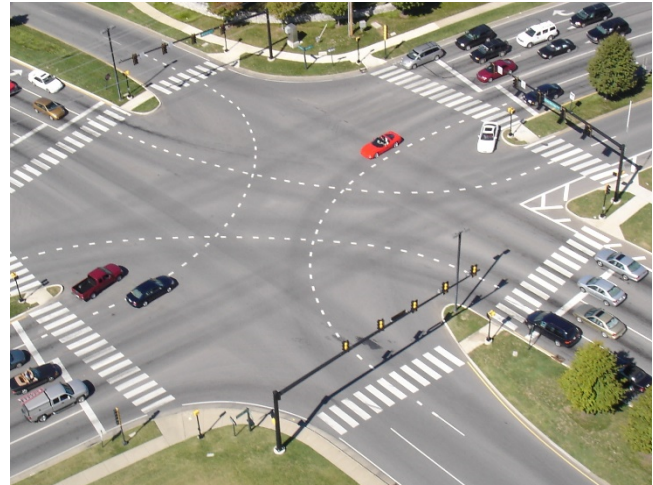
Channelization at intersection
