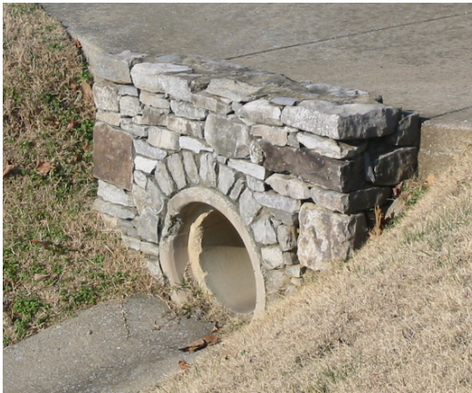
Protected Endwall with Stone Veneer
