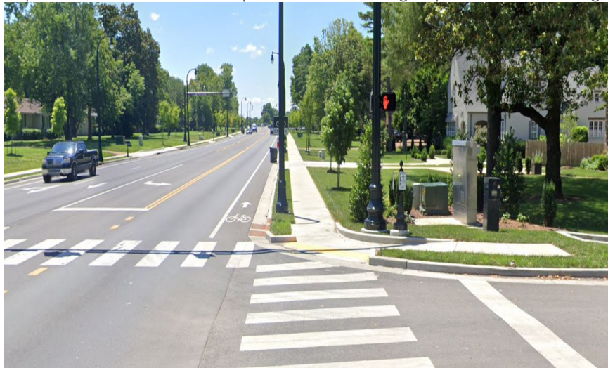
Existing bicycle lane on Hillsboro Road.
