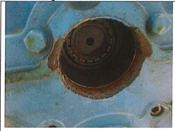
Picture #4: High speed cover on non-input side is damaged
