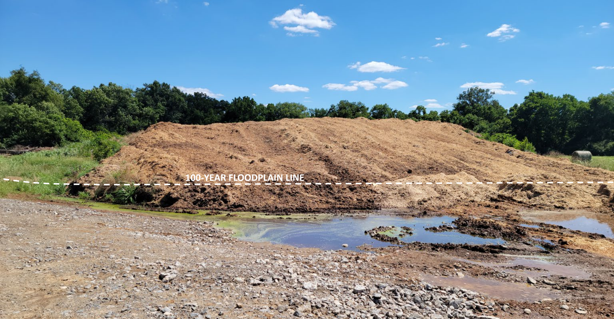
EXISTING MUCKED STALL DISCARD AT SOUTH END OF PROPERTY
