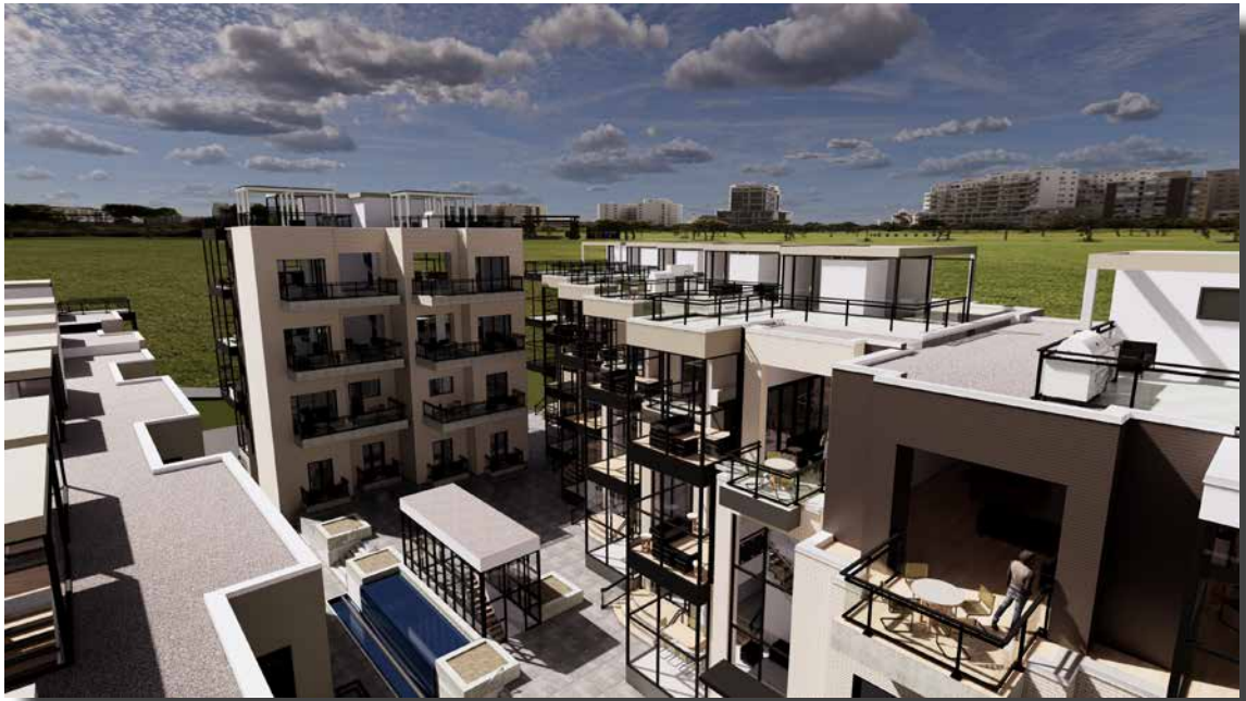
View from courtyard toward Cool Springs Blvd
