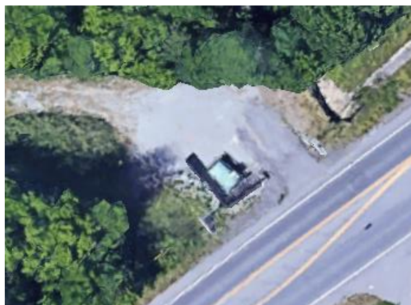
Figure 7 - Carters Creek Pike PS Aerial View
